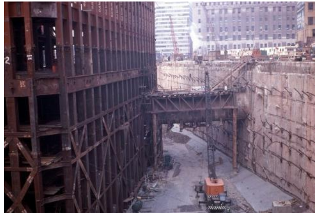
WTC Slurry Walls & Tiebacks
