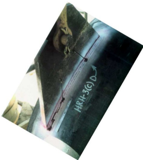
Fig 1. A horizontal and vertical dummy leg installation that cannot be accurately analyzed due to unknown effect on the elbow flexibility, and the unknown interaction of the SIF's.
