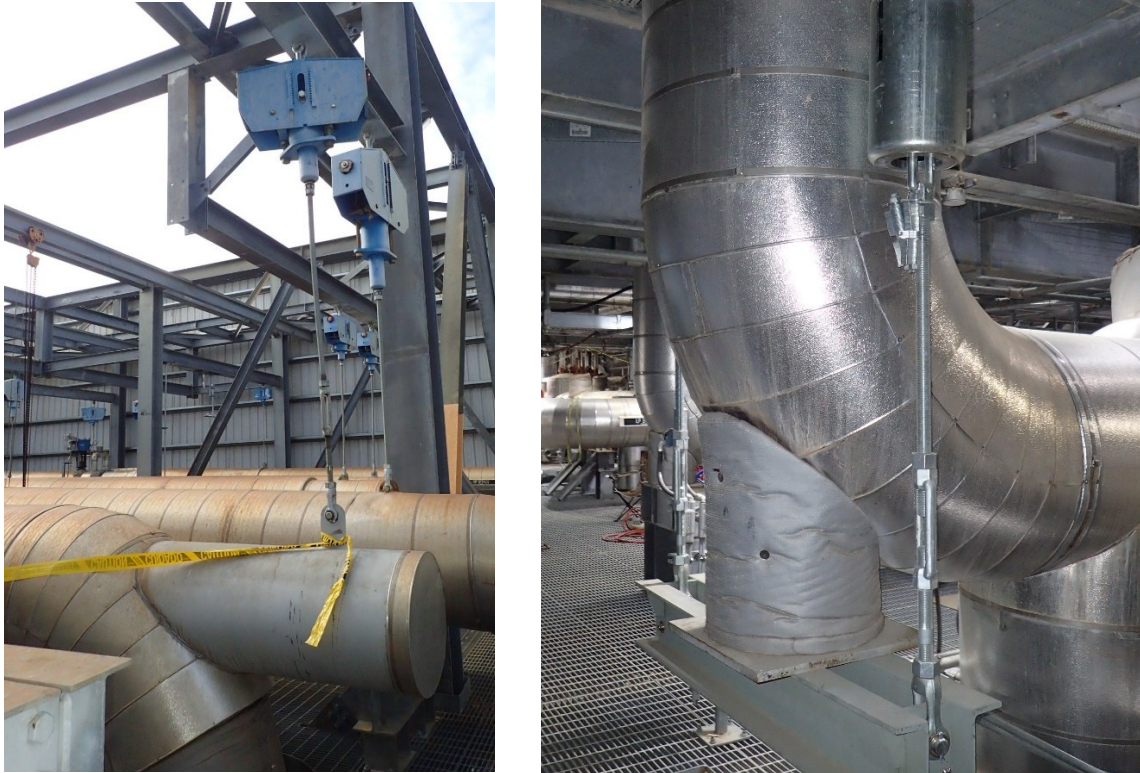
Fig 1. A horizontal and vertical dummy leg installation that cannot be accurately analyzed due to unknown effect on the elbow flexibility, and the unknown interaction of the SIF's.
