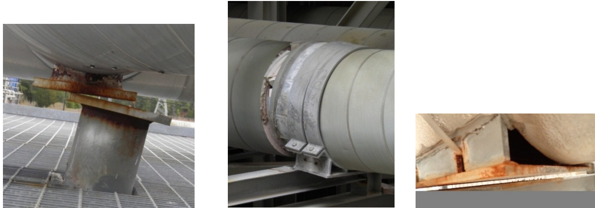
Figure 7. When sliding supports rotate off of flat on flat, there is no data for the friction factor. While the left two photos are dramatic, the right photo is typical in the field of a slight rotation in which only part of the slide plates are touching. The perpendicular forces are concentrated in a small area leading to possible gouging of the slide plates. Analysis would miss this problem completely.
