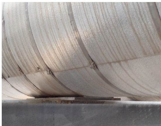
Figure 7. When sliding supports rotate off of flat on flat, there is no data for the friction factor. While the left two photos are dramatic, the right photo is typical in the field of a slight rotation in which only part of the slide plates are touching. The perpendicular forces are concentrated in a small area leading to possible gouging of the slide plates. Analysis would miss this problem completely.
