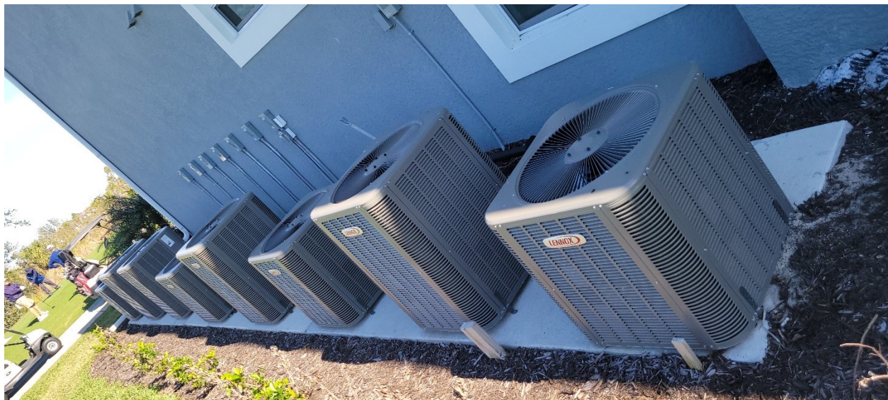
Cast-in-place pad at grade level with expansion joints
