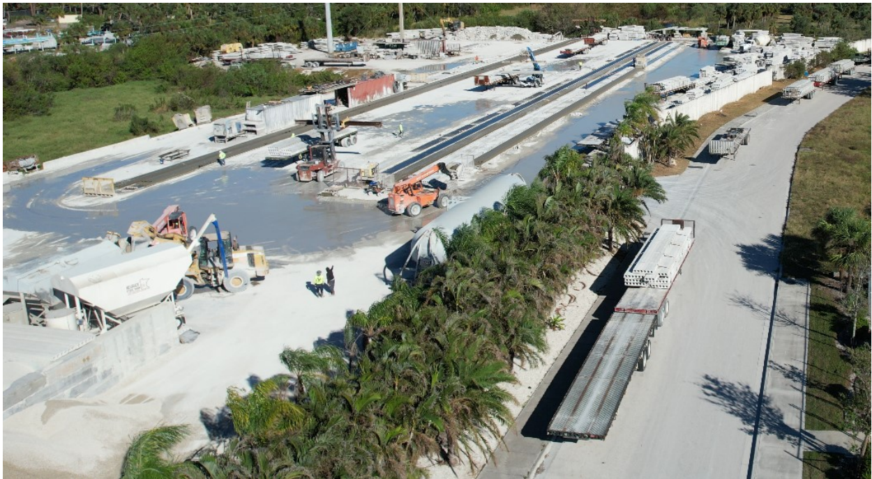
A precast concrete plant operation
