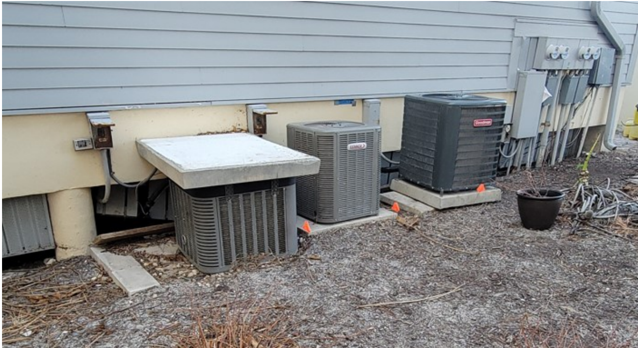
Blue tape just below the siding marks proposed condenser underside elevation.
