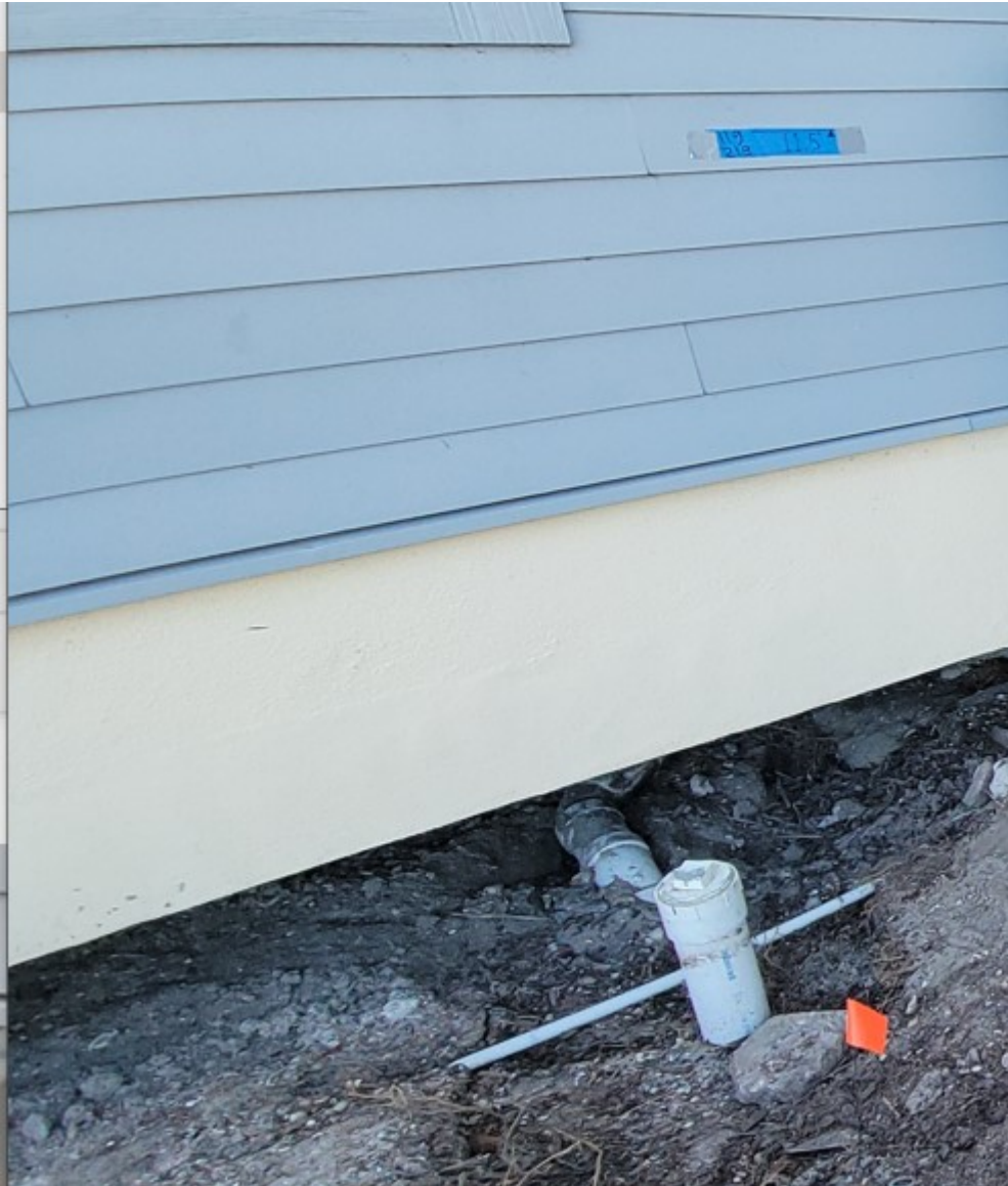
Blue tape marks required elevation at 11.5 ft in 10 ft flood zone
