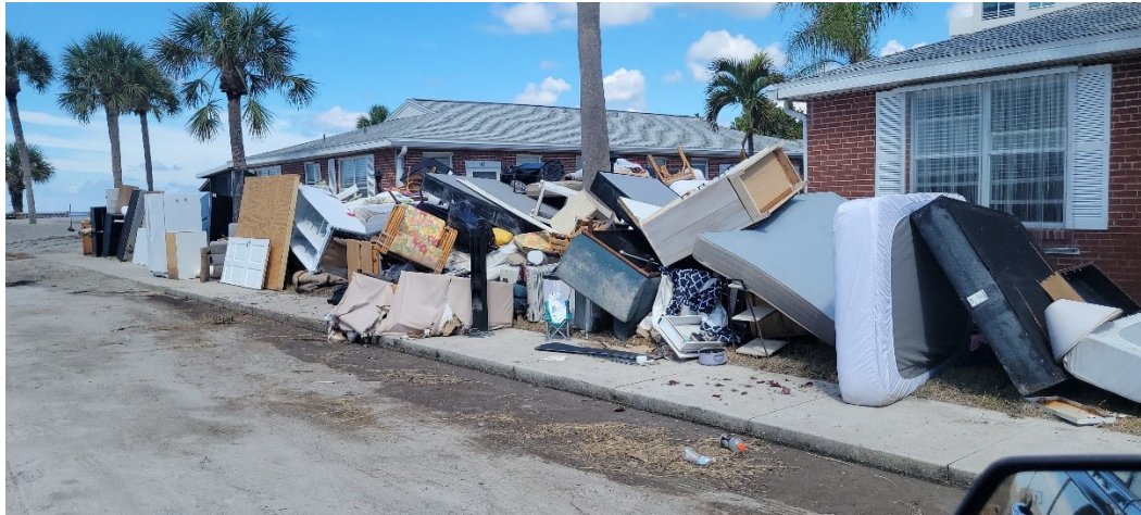
Non-conforming structures with first floors below the flood plain level and freeboard.
