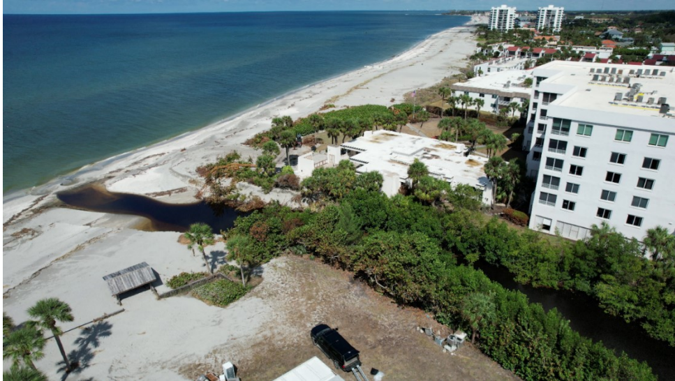
Drainage channel outfall that is part of a network of swales and pipes draining into it.
