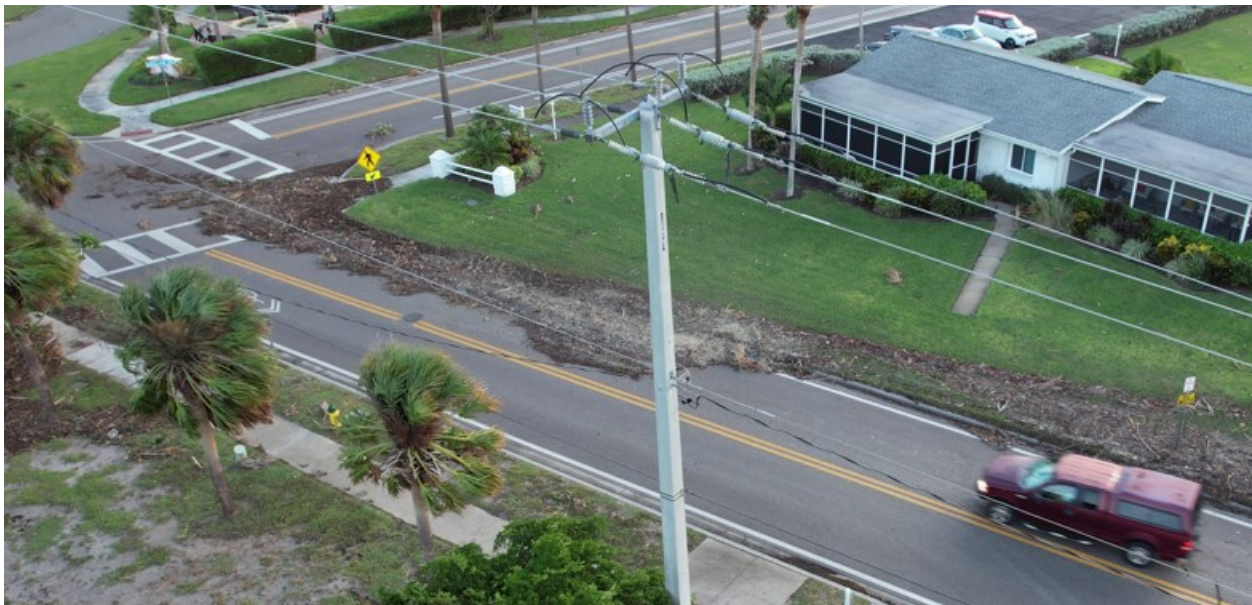
Roadway debris from a flood event
