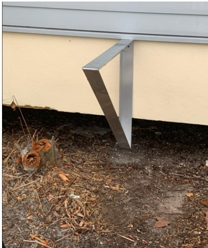
Proposed bracket screwed into concrete floor beam
