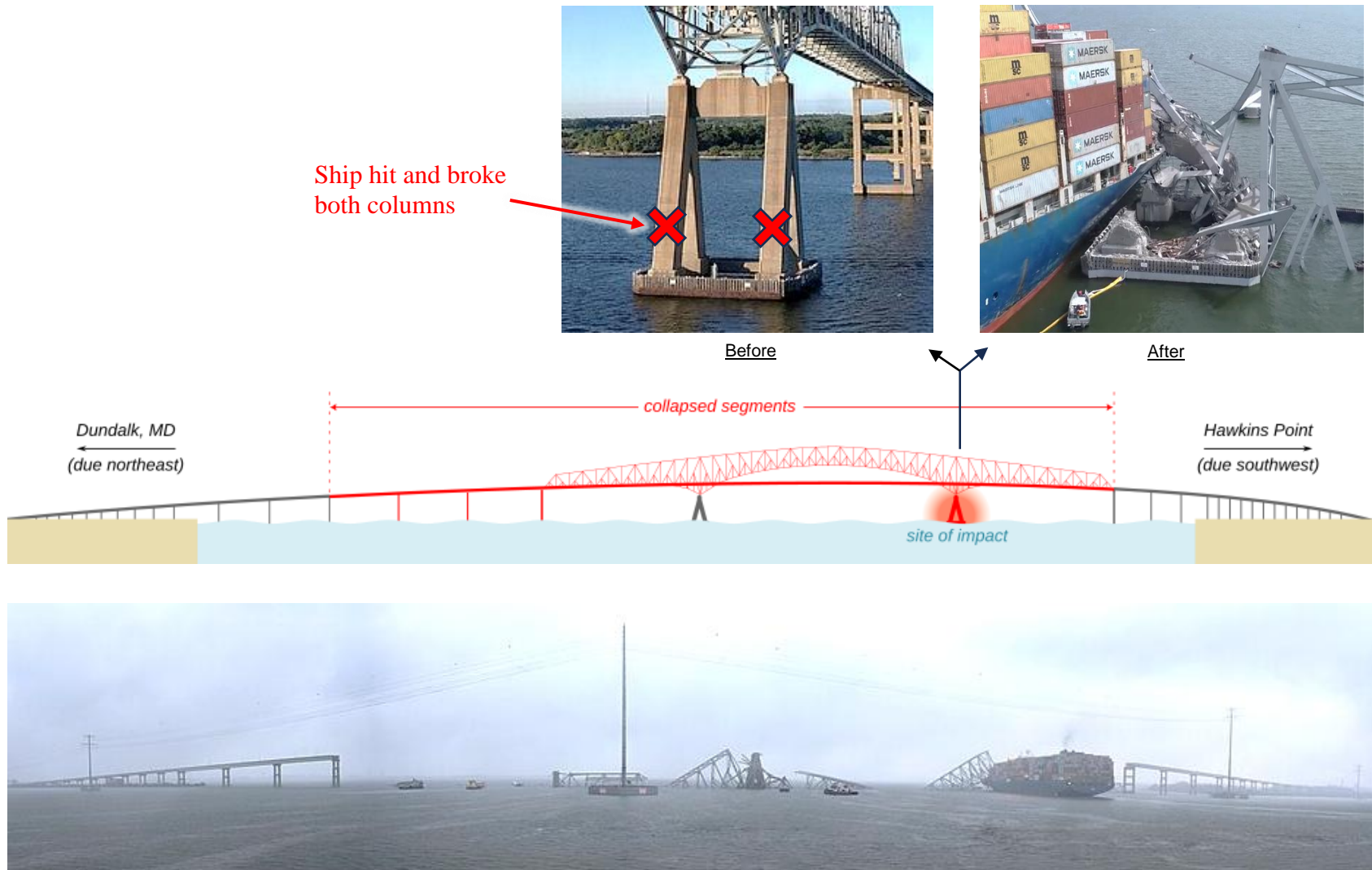
Figure 2: Views looking southeast with collapsed portion of the bridge in red.
