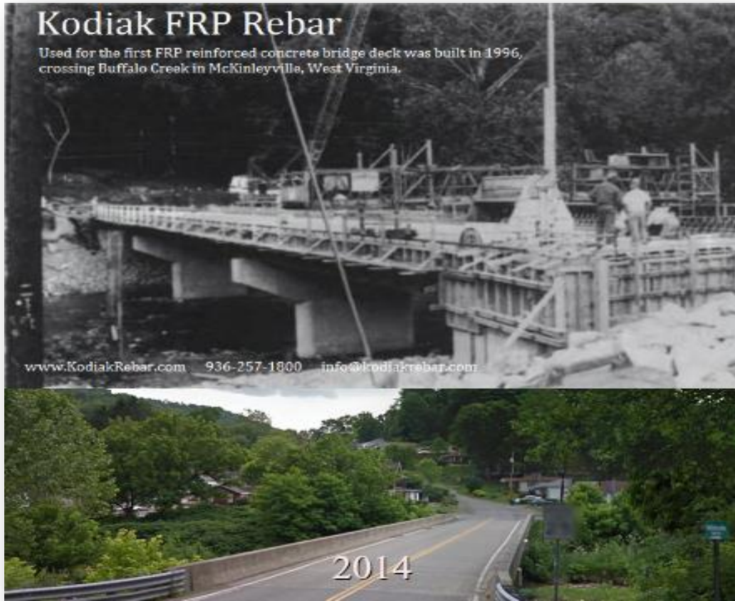
Kodiak Fiberglass Rebar, used for the First FRP Reinforced Bridge in U.S. History (Mckinleyville Bridge over Buffalo Creek, West Virginia 1996)
