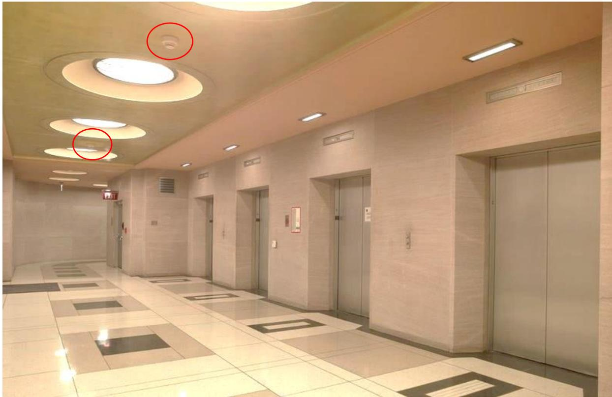
Figure 14: Elevator lobby with smoke detectors circled in red.
