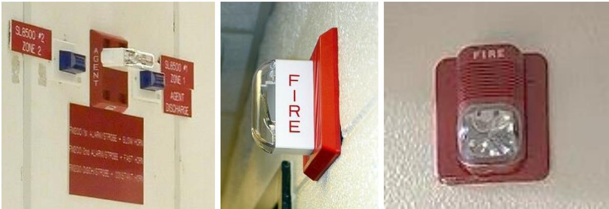
Figure 6: Example audible and visual fire alarm devices.
