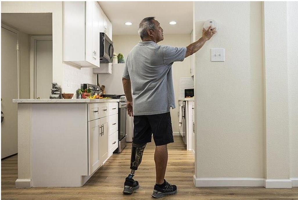
Figure 11: Smoke alarm near a stove (cooking appliance).
