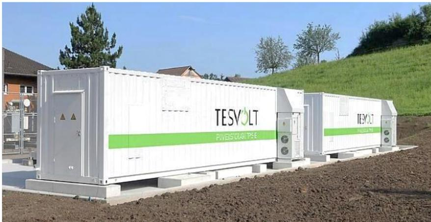
Figure 2: A 6 MWh battery storage power station may be exempt from needing an automatic sprinkler system per 2024 IBC 903.2, unless it has lithium-based batteries.
