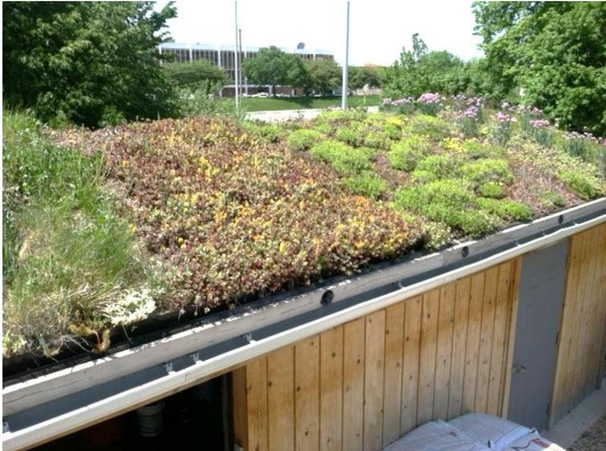
Figure 9: Example vegetative roof (green roof).
