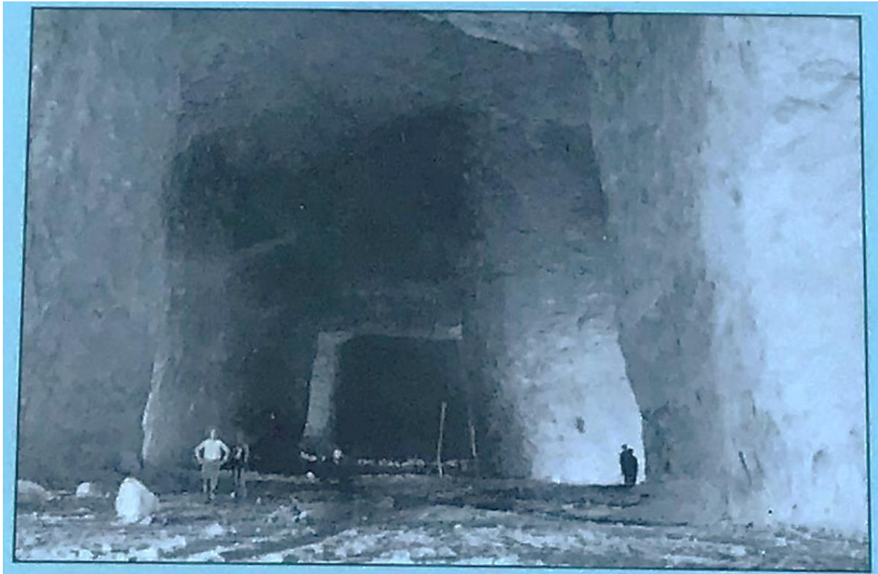
Figure 2: Picture from inside the salt mine below Lake Peigneur prior to the disaster. The salt pillars were left to help hold up the ceiling of the mine.
