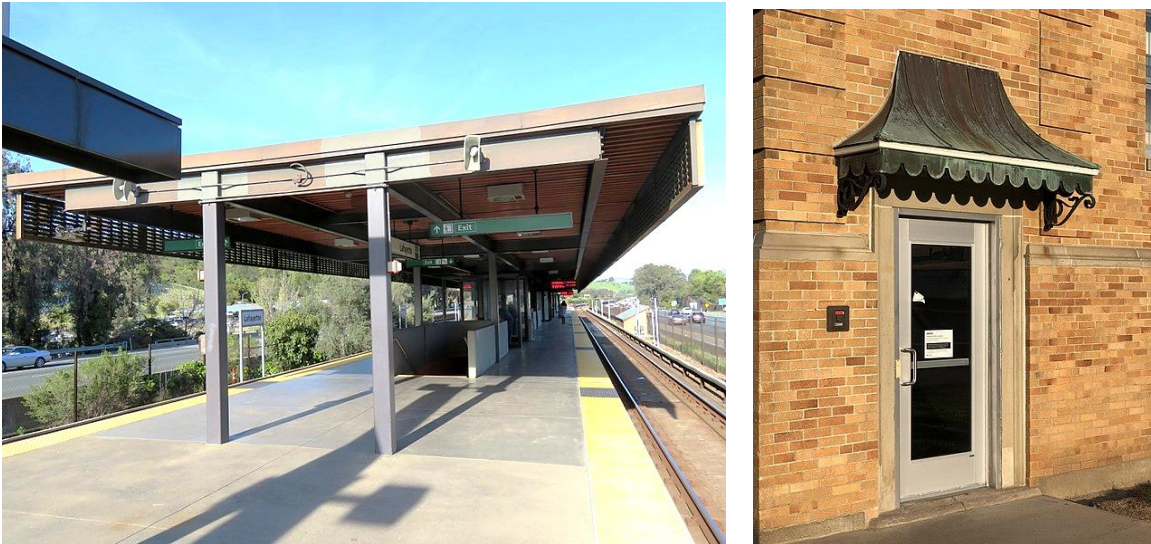
Figure 11: Example self-supporting canopy (left) and awning/marquee (right).
