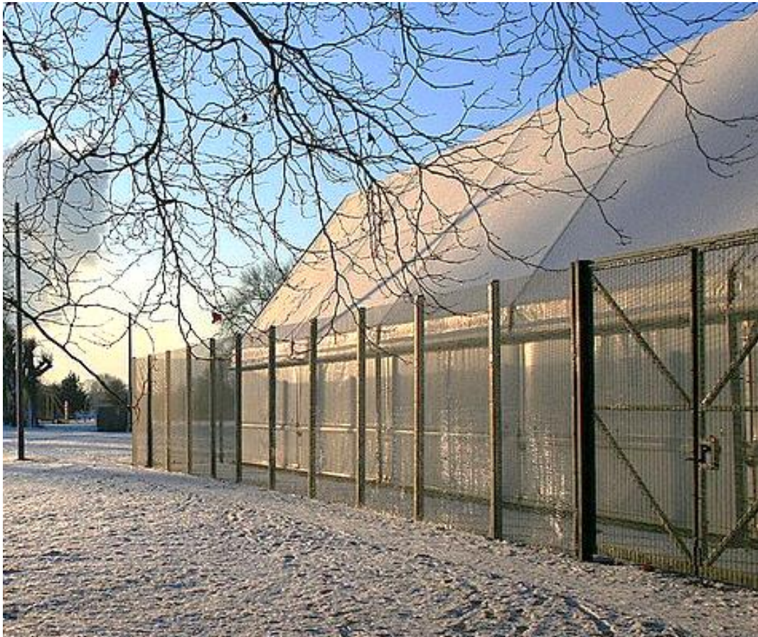
Figure 14: Example temporary structure.
