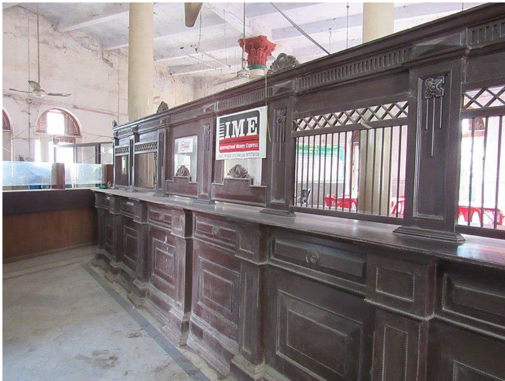
Figure 7: Example partition wall (non-load bearing wall).
