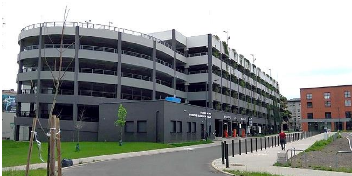
Figure 5: Example of a freestanding parking garage.
