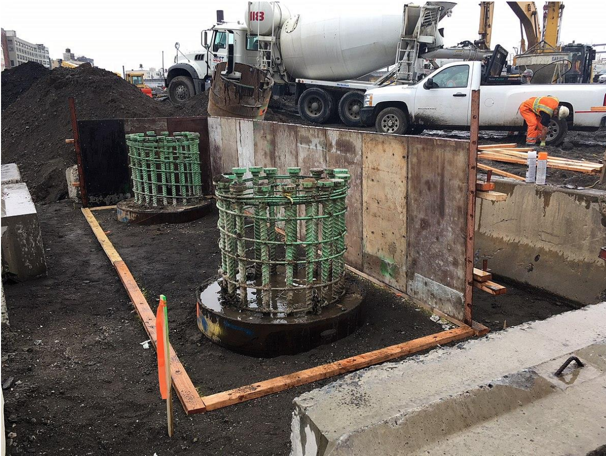
Figure 9: Installing forms for a cast-in-place pile cap on two piles.
