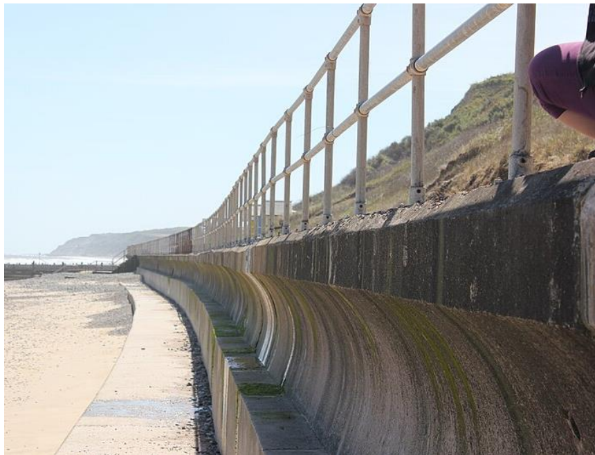
Figure 2: Example of guardrail on a retaining wall.
