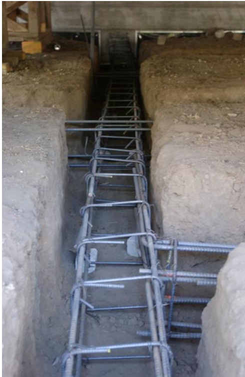
Figure 10: Reinforcement for cast-in-place grade beams.
