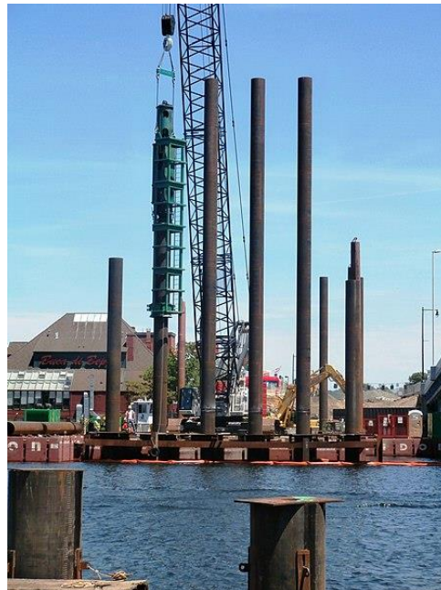
Figure 11: Depiction of vibratory driving (left) and example installation (right).
