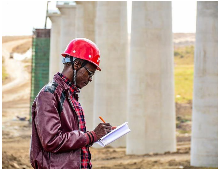
Figure 4: Special inspector writing field notes for concrete pier installations.
