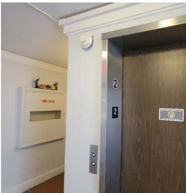
Smoke alarm noted.
