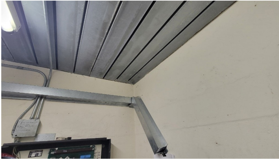
Load bearing walls beneath Q deck.
