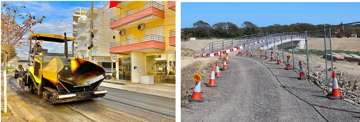
Figure 4: Road construction capital improvement projects.
