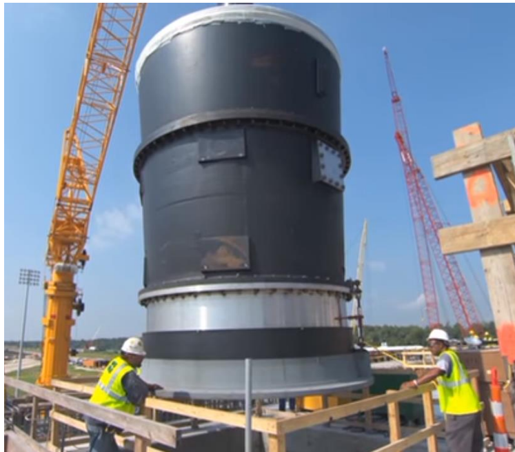
Figure 1a: Left: Author next to the top of a large vertical pump for moving canal water. Right: The lower section of an 11' dia. vertical pump for flood protection.
