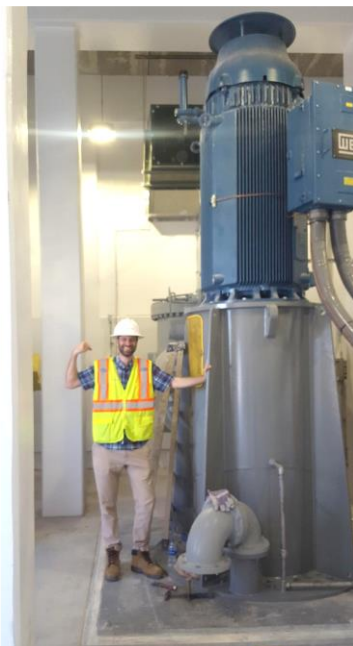
Figure 1a: Left: Author next to the top of a large vertical pump for moving canal water. Right: The lower section of an 11' dia. vertical pump for flood protection.
