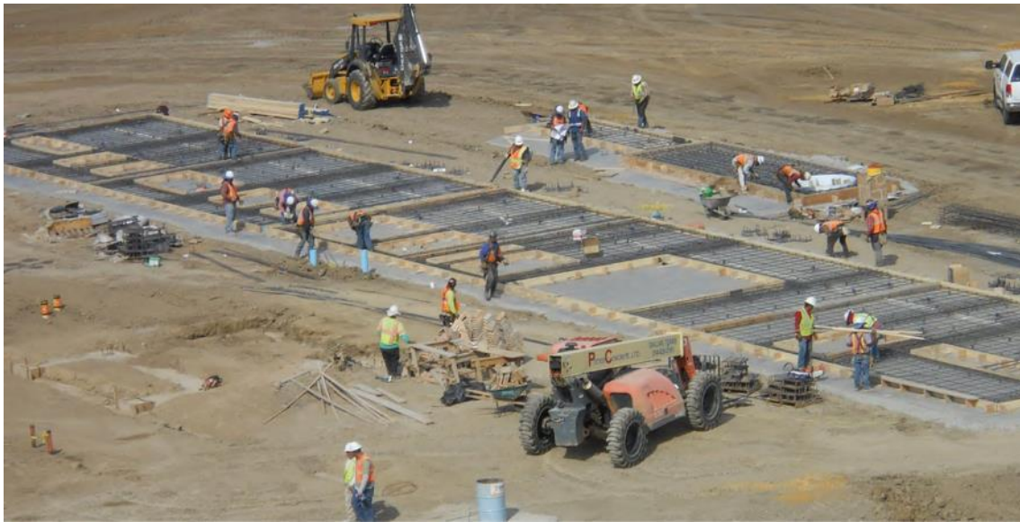
Fig. 3, Separate panels being prepared for pour with reinforcement in place
