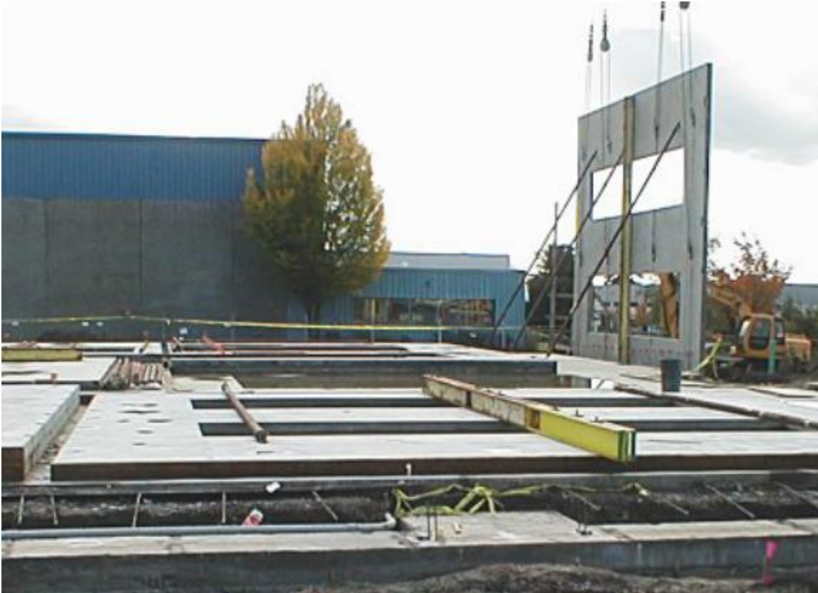
Fig. 41: Strongbacks attached to panels
