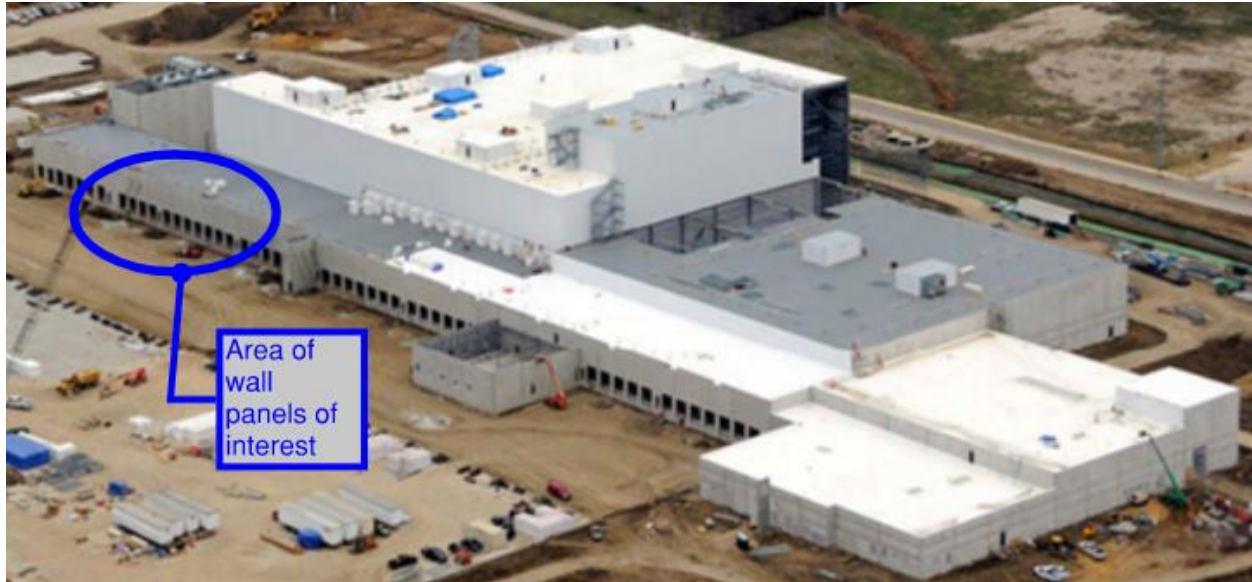
Fig.15: Aerial view of facility with tilt-up wall panels
