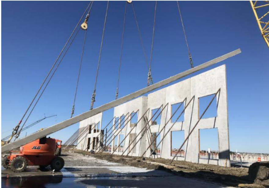
Fig. 5a, Panel being picked by crane rigging
