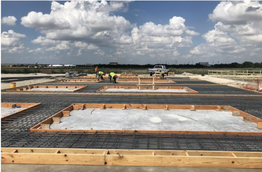
Fig. 37: Wood forms for tilt-up panels
