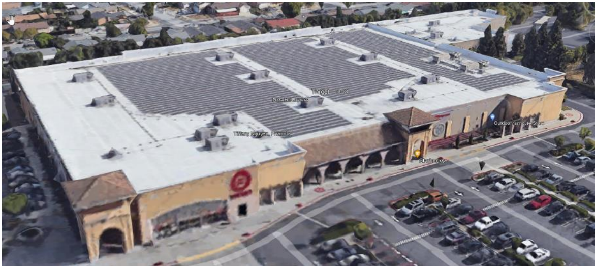
Fig. 8. Retail store in San Jose, CA, with tilt-up wall panels (Google Earth)
