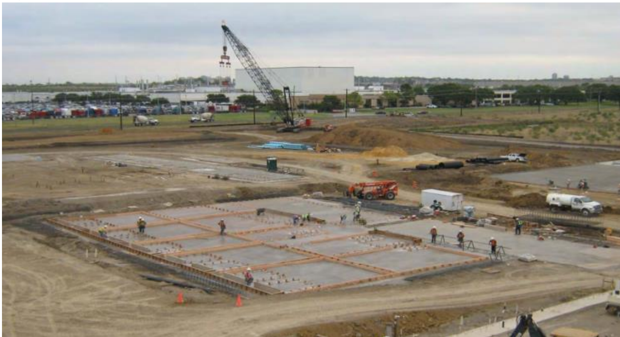
Fig. 48: Lay down area
