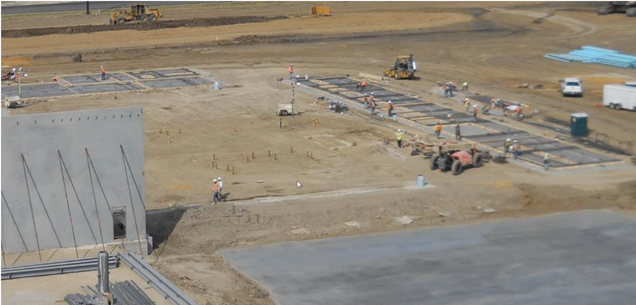
Fig. 35, Sequenced panel construction:
