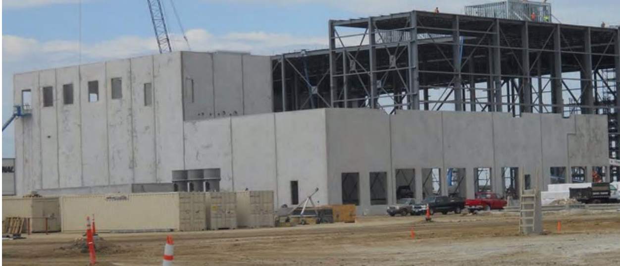
Fig. 2, Erected tilt-up panels placed side-by-side
