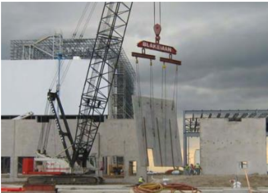
Fig. 5b, Crawler crane moving a panel
