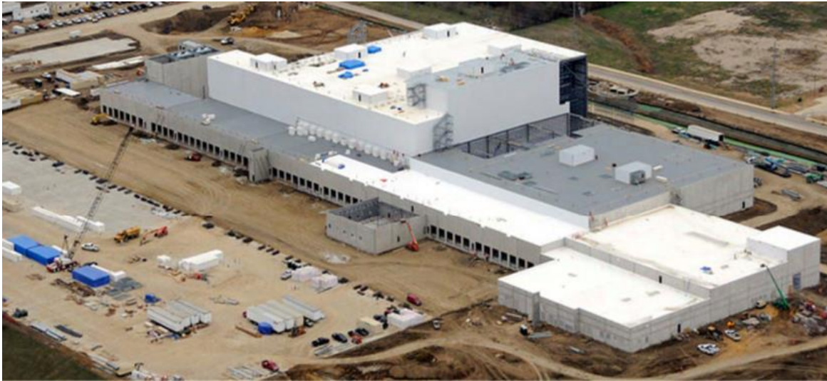
Fig. 1 - Progress photo of a project with tilt-up concrete walls
