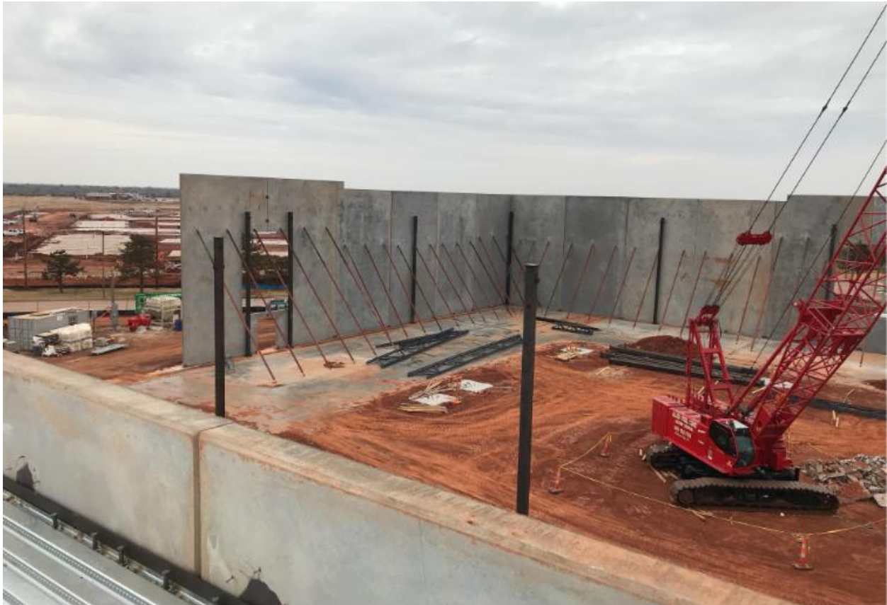
Fig. 7: Wall panels with diagonal braces to ground
