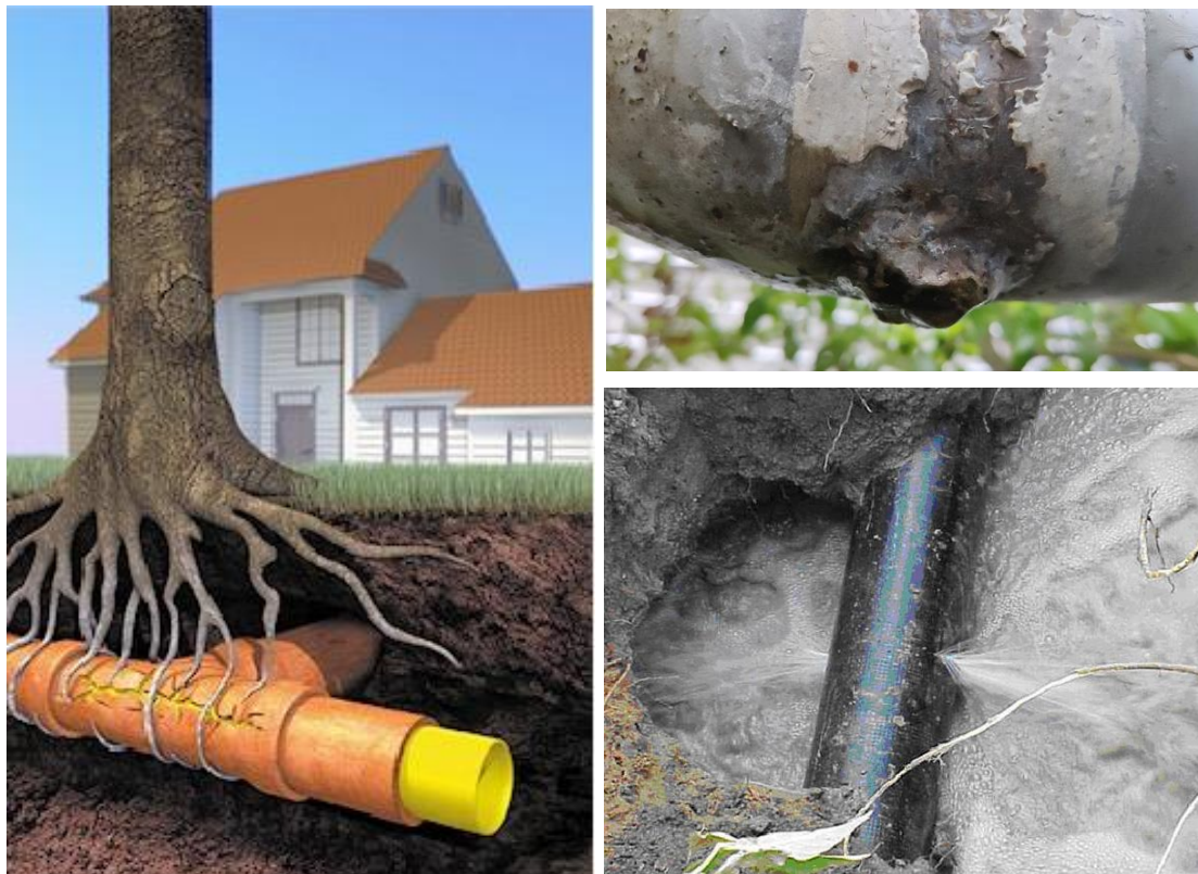
Figure 13: Left: tree roots stressing a pipe. Upper right: Slow leak at a defect in a joint. Lower right: Large leak on a water main with an unknown cause.
