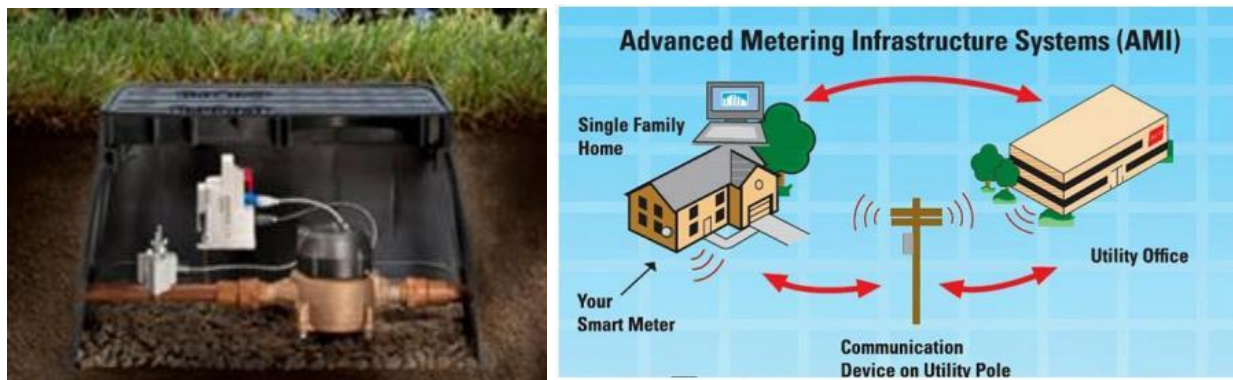
Figure 9: Left: Water meter with AMI communications device in white. Often these radio communications devices will look like hockey pucks on the lid of the meter box. Right: Basic components of an AMI communications system.
