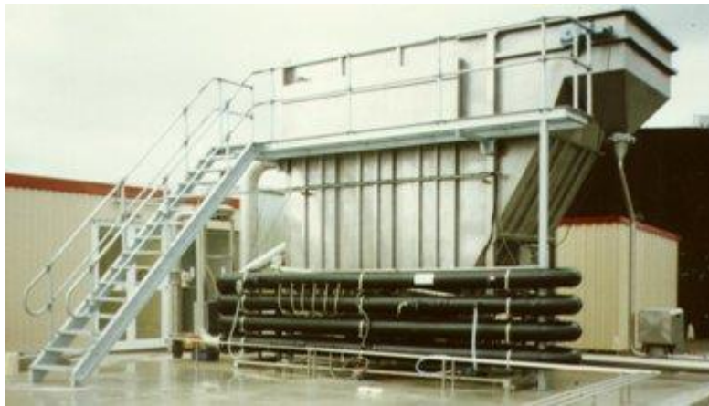
Figure 6: Example of a dissolved air flotation pretreatment system. These are common at oil refineries, chemical plants, and paper mills.
