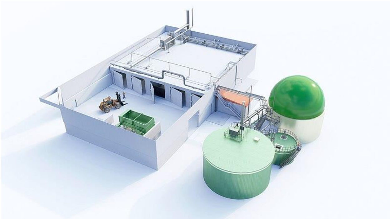
Figure 3: Example of a large industrial pretreatment system with secondary treatment and digestion.
