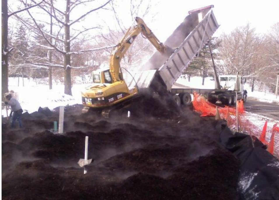
Figure 11: Wood chips being poured on top of the stone plenum to form the media bed.
