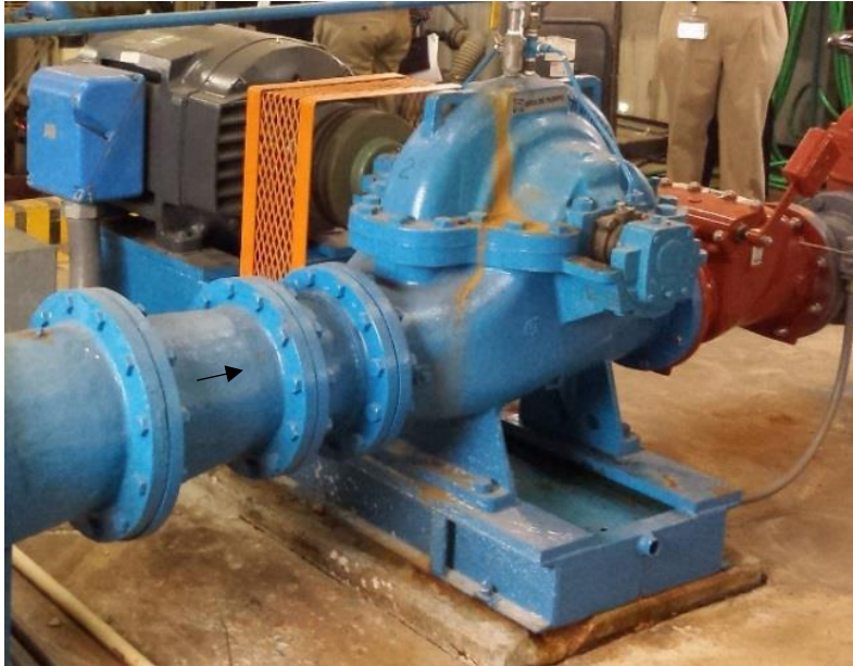
Figure 4: A horizontal split-case centrifugal pump for finished water pumping. Flow enters on the left and splits to either side of the impeller. The impeller receives flow in the center from both sides and discharges to the right.
