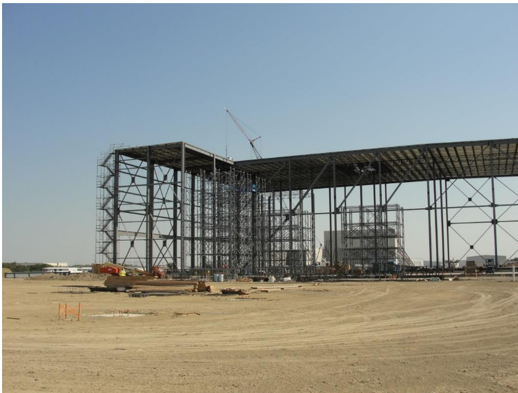
Fig. 39, Roof-supporting storage racking being placed adjacent to conventional steel-framed warehouse structure
