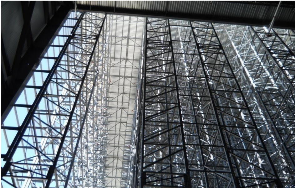
Fig. 38, Storage racking that supports the roof and braces the wall panels
