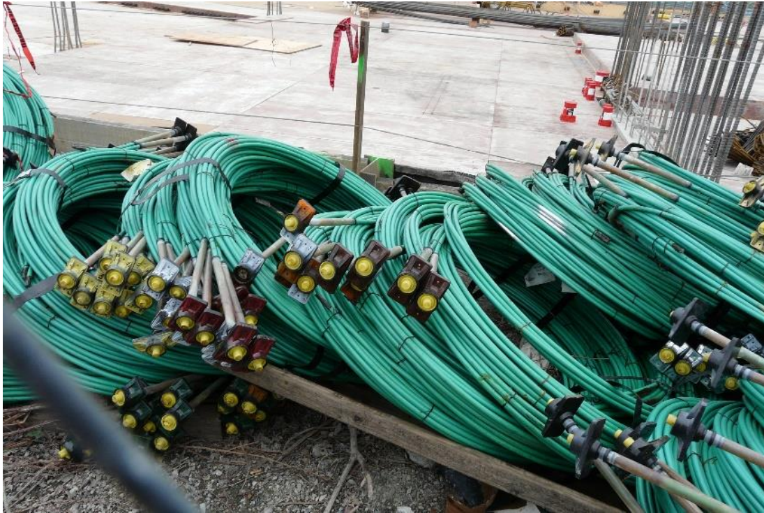
Fig. 22, Post-tensioning tendons ready to be placed
