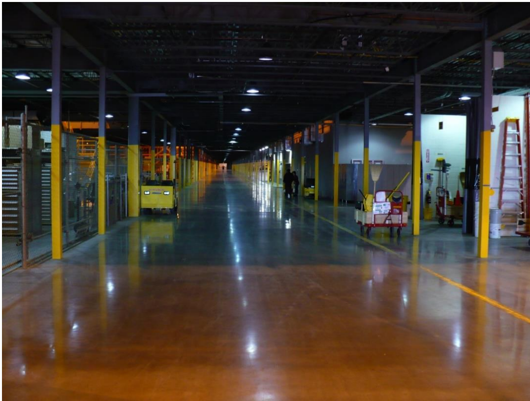
Fig. 18, Continuously reinforced high speed travel aisle
