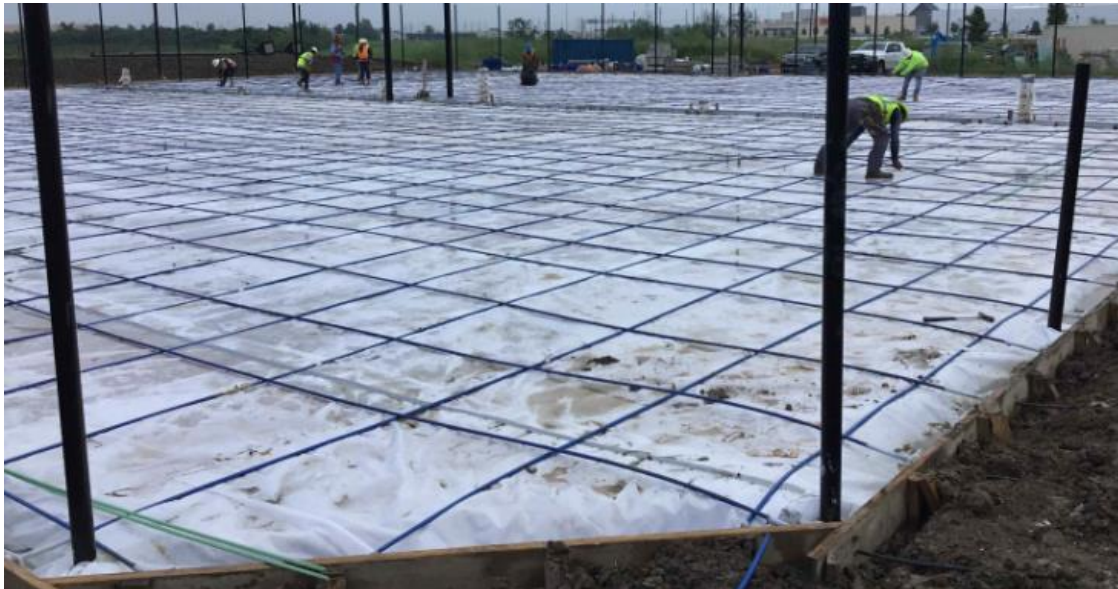
Fig. 23, Post-tensioning tendons in place over poly
