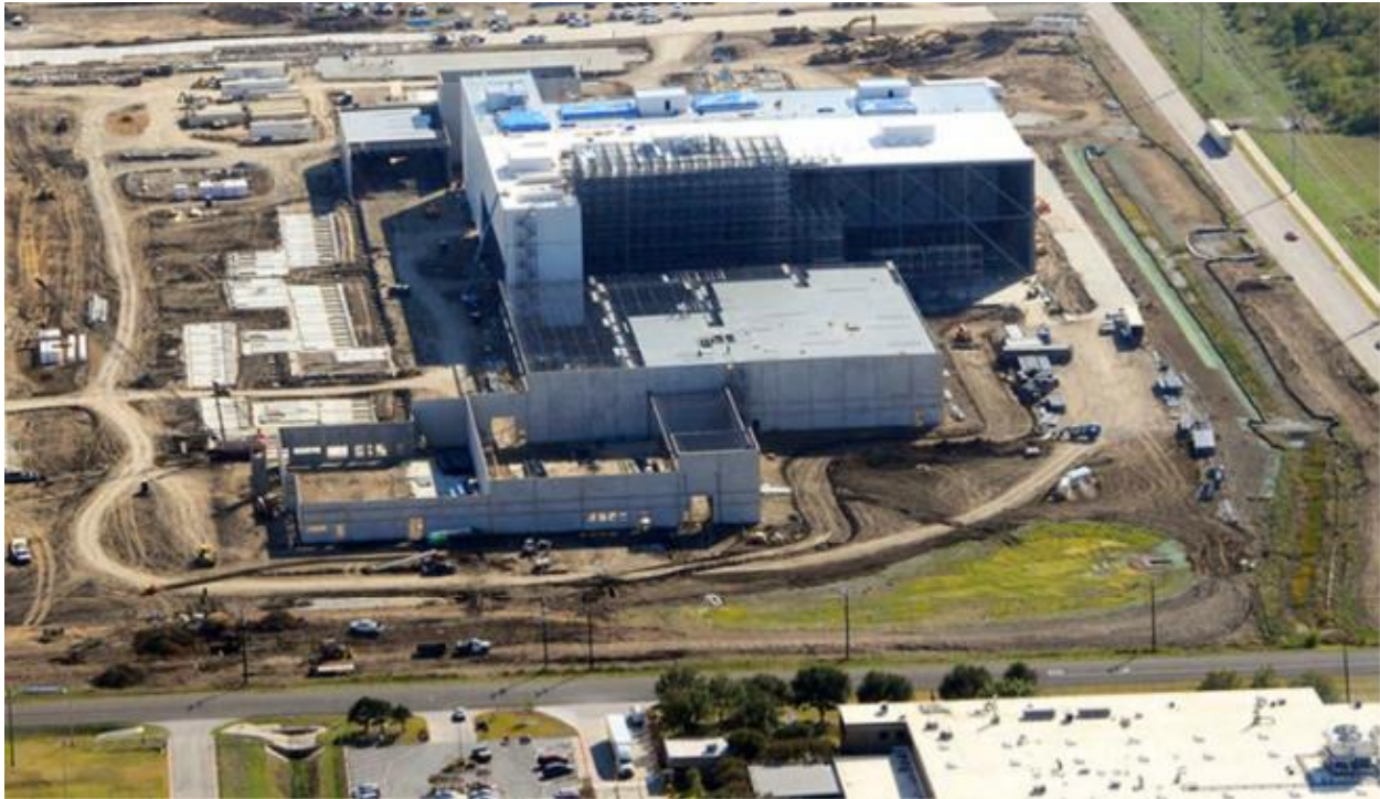
Fig. 40, Roof-supporting storage racking being placed adjacent to conventional steel-framed warehouse structure
