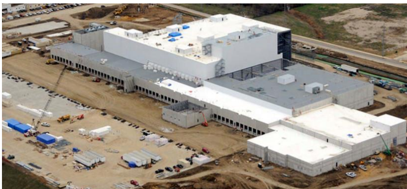
Fig. 1 - Computer rendering and progress photo of a refrigerated food warehouse
