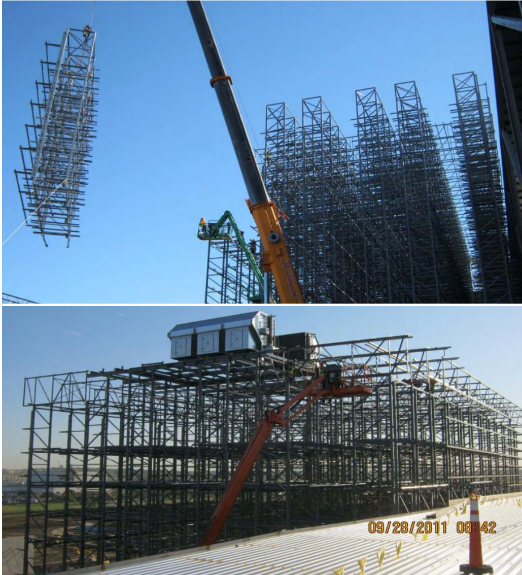
Figs. 43 & 44, Racking that supports the roof and braces the walls
