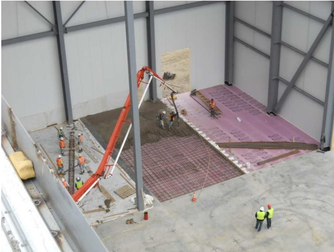
Fig. 34, Freezer slab being poured
