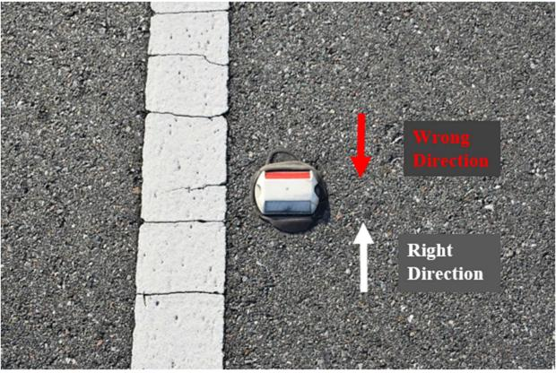
Figure 10. Bidirectional raised pavement marker depicting right and wrong directions of travel
