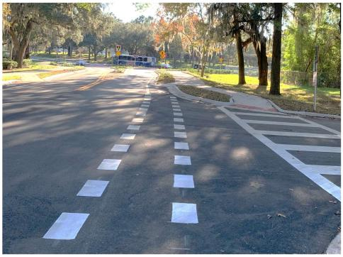
Figure 9. Dotted-edge line for bike path across driveway access point
