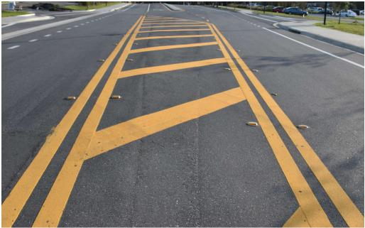
Figure 20. Crosshatch marking
