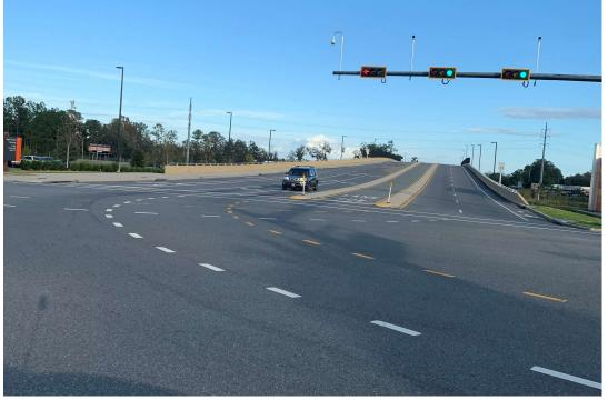
Figure 8. Dotted-edge lines extended through intersection
