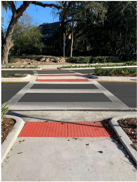
Figure 33. Pedestrian detectable warning surfaces
