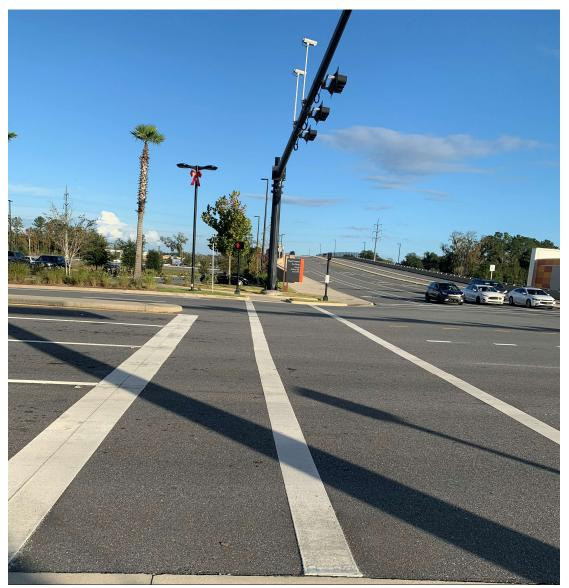
Figure 15. Transverse markings of stop line and crosswalk
