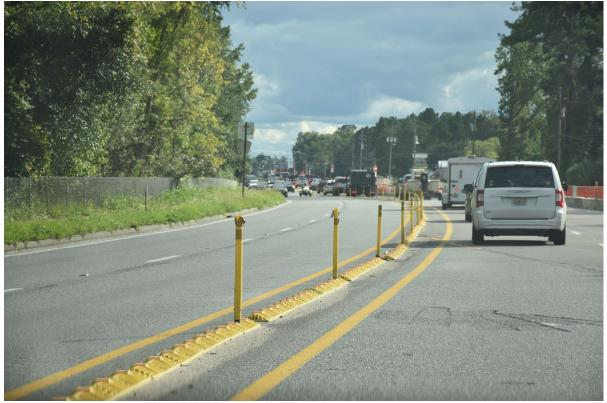
Figure 30. Center line channelizing devices
