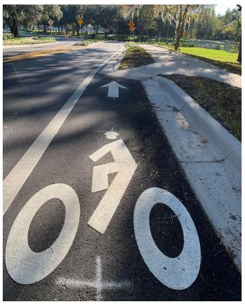
Figure 22. Bicycle lane roundabout termination
