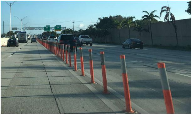
Figure 31. Lane divide channelizing devices
