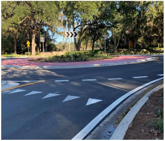
Figure 21. Roundabout approach marking
