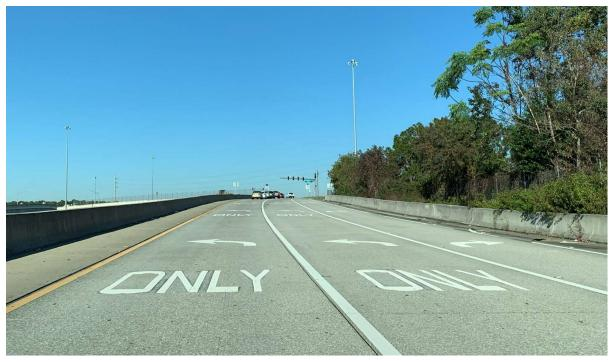
Figure 18. Word and arrow pavement marking
