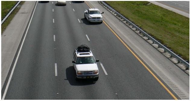
Figure 34. Longitudinal rumble strip with edge line not on rumble strip
