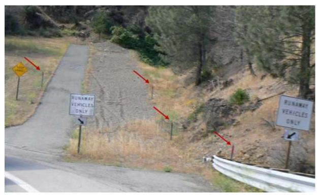
Figure 27. Truck escape ramp with red post-mounted delineators
