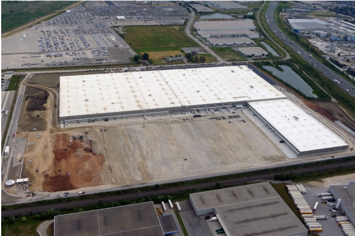
Aerial View of Warehouse Site with Building Shell Nearing Completion
