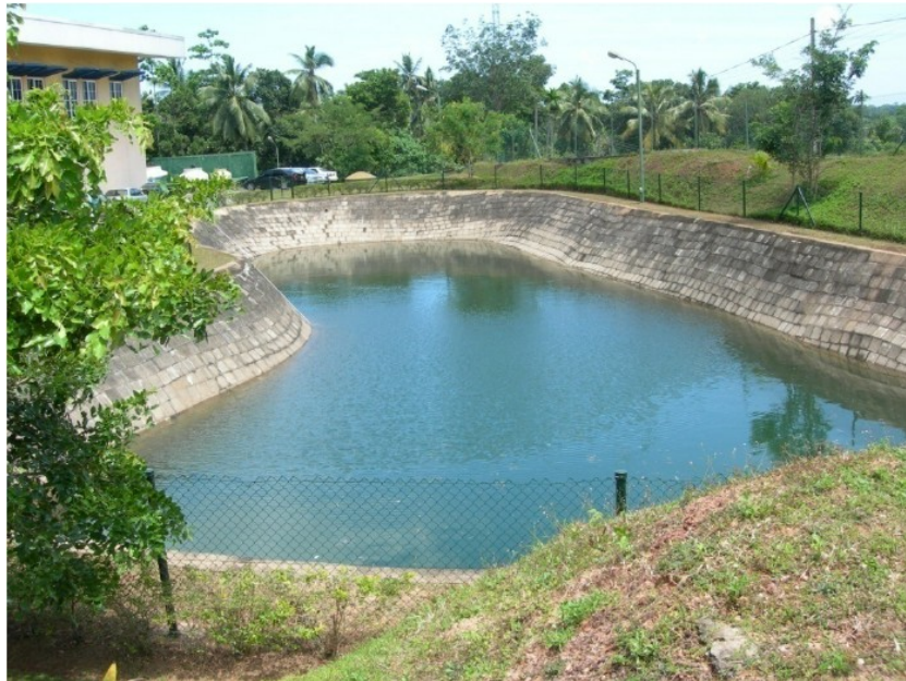
Figure 17: Example of a rainwater storage tank.
