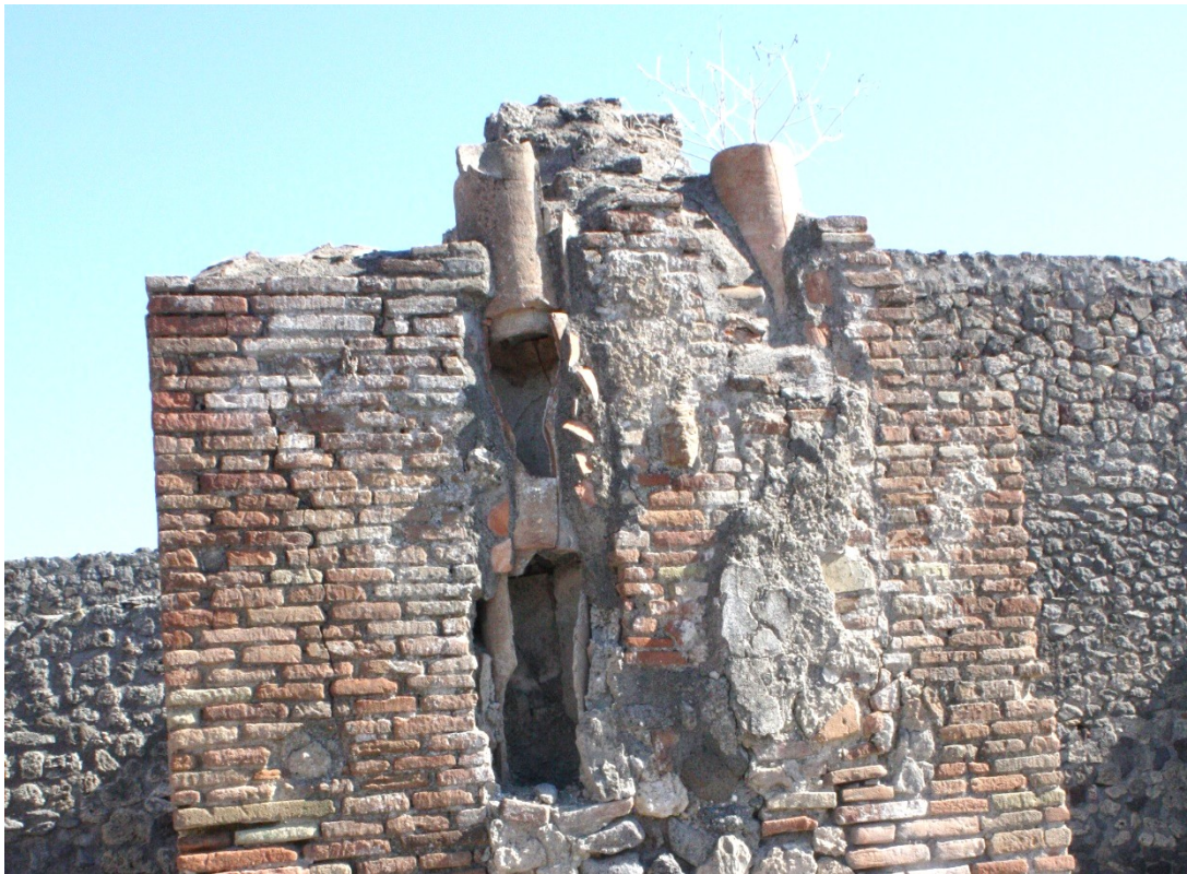
Figure 2: Ruin of a Roman-era building in Pompeii with sewer pipes seen in the walls. The pipes carried wastewater down to larger collection pipes below the street.
