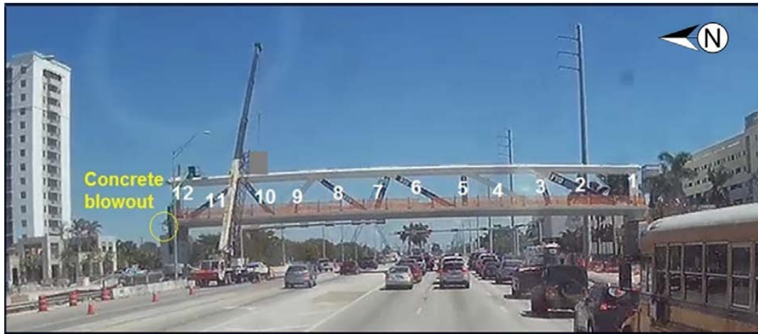
Figure 9 – Still frame from in vehicle video showing concrete dust and debris blowout at node end of main span north of node 11/12.
