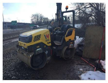
Low Profile Rollers and Mechanical Plate Tampers: Low Clearance for Bridge Reconstruction Projects, The lightweight doesn't displace the CMU facing blocks while compacting the backfill lifts.
