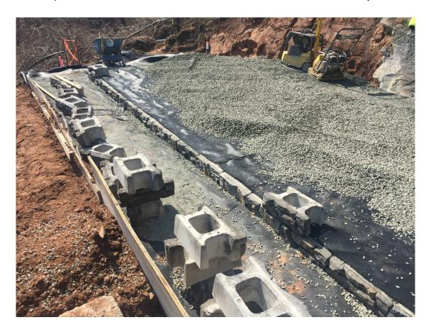
Regardless, any overlap at the CMU must be trimmed to avoid varying fabric thickness under the blocks which will cause instability. Place aggregate backfill in a constant direction making sure not to shift the geotextile fabric and cause wrinkles or tears. Stagger seams by a minimum of 2 feet with each successive lift of aggregate/geotextile backfill.
