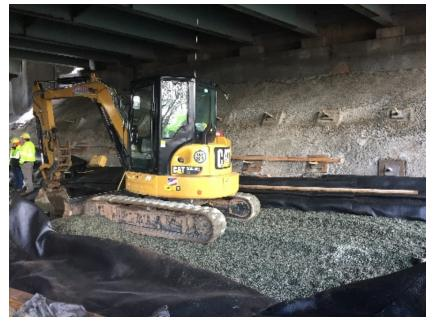
Mini-Rubber Tracked Excavators and Mini-Mini-Rubber Tracked Excavators: Low clearance and maneuverable. For spreading and grading aggregates. The low profile is helpful on bridge reconstruction projects. Rubber Tracks allow for load distribution on and movement on loose graded No. 8 & 67 aggregate.
