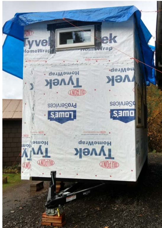
Installed Tyvek Home Wrap used as a water-resistive barrier (WRB)
