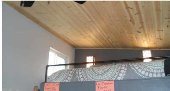
Gypsum board (drywall) walls in a THOW
