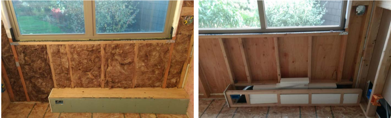
Left: Fiberglass roll insulation in the walls of a THOW
