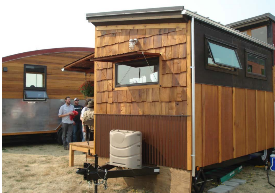
THOW (in foreground) using multiple siding materials including painted corrugated steel panels, cedar shingles, Breckenridge siding panels, and faux board and batten siding
