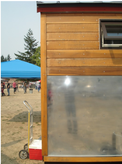
Left: THOW using tongue and groove wood siding and sheet metal for siding
