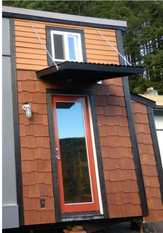
Removable, adjustable awning supported by hinges and chains
