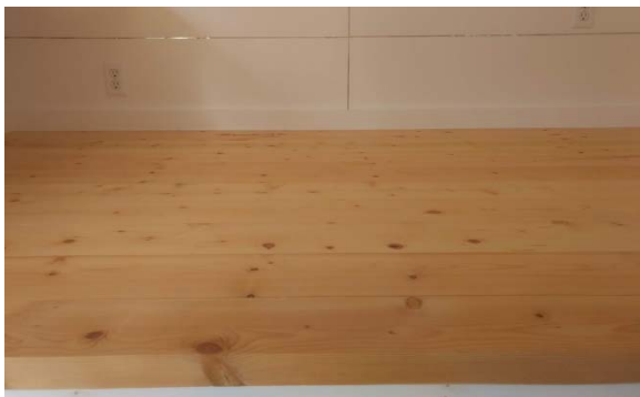
Left: Wood 2x6 decking for loft flooring in a THOW
