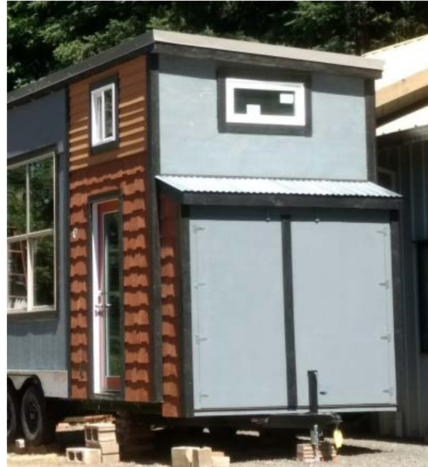
Two examples of THOW exterior storage cabinets
