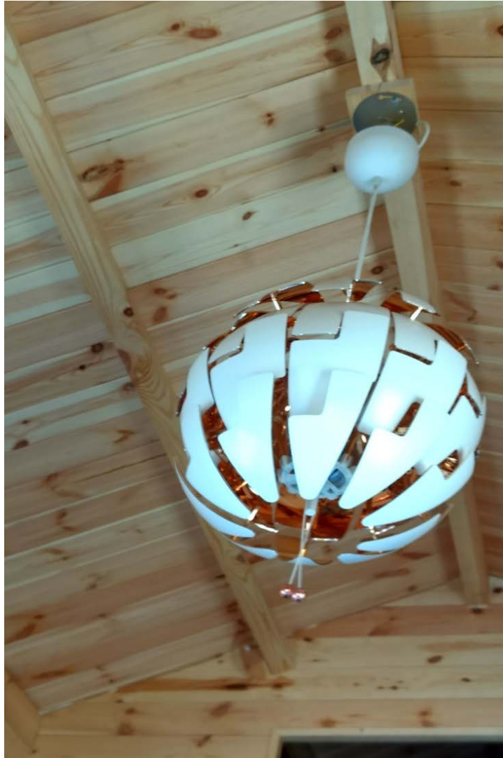
Exposed roof framing members with tongue and groove lumber roof sheathing
