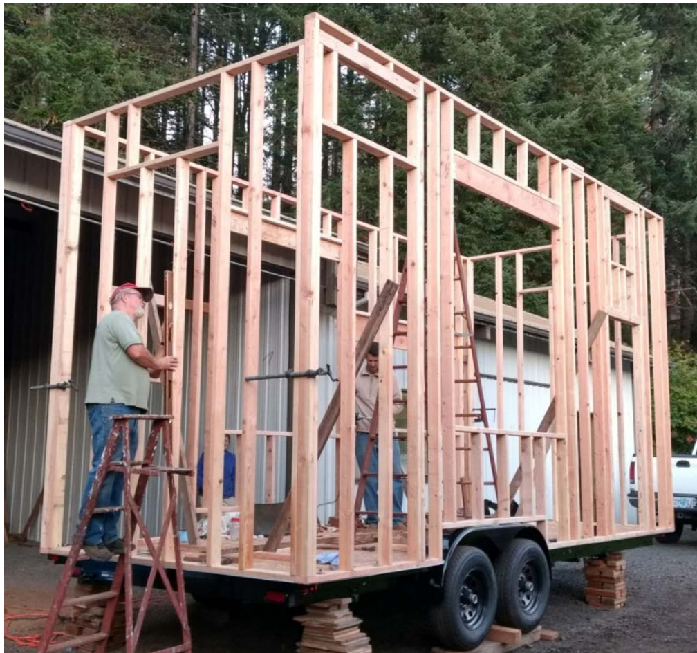
Straightened, leveled, and plumbed THOW framed walls
