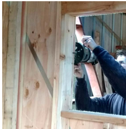
Coiled metal strapping (Simpson Strong-Tie CS-22) running diagonally between studs
