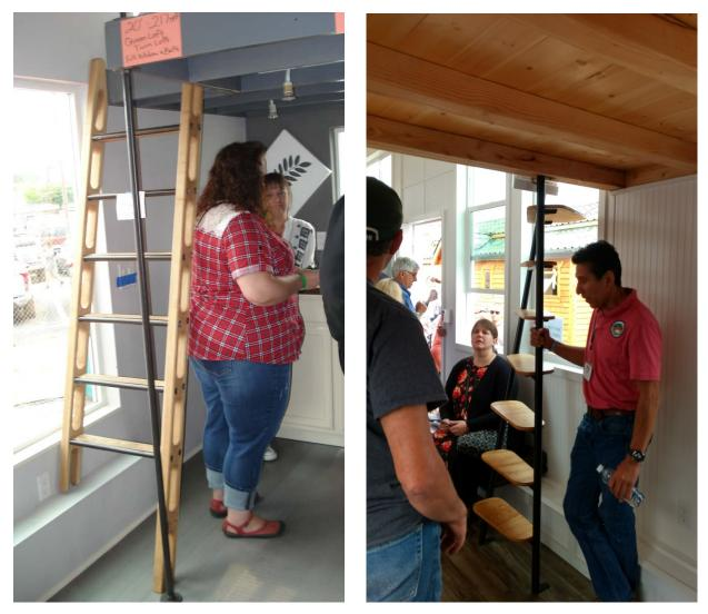
Left: Loft ladder with one leg standing on a framed out wheel well Right: Spiral loft ladder with custom metal frame to take up less floor space
