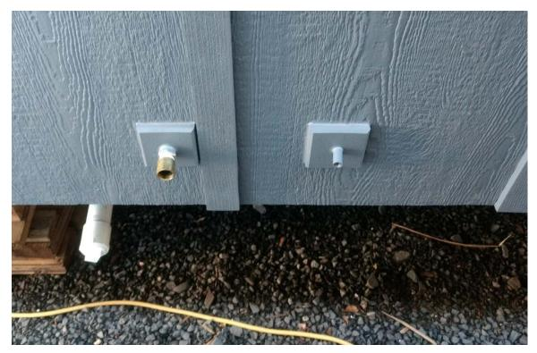
From Left to Right: Gray water discharge connection for sink, potable water hose connection, potable cold water drain outlet used for winterization of this THOW
