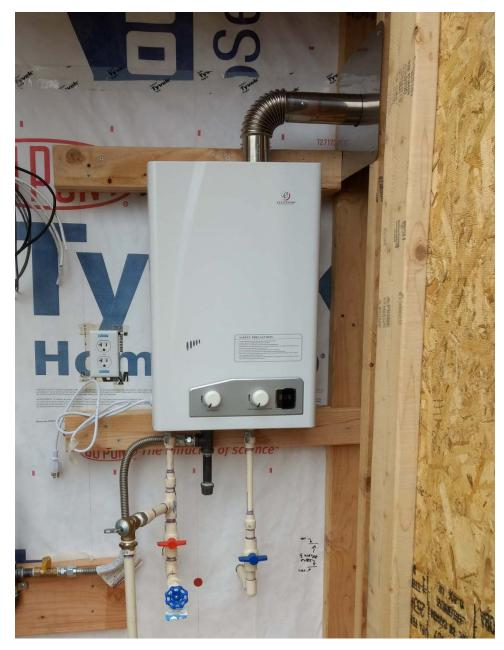
A tankless, or on-demand, propane hot water heater installed in a THOW. Notice the vent coming out the top of the unit. This water heater model plugs into a 120 volt electrical receptacle to power the flame igniter. Models with battery powered flame igniters are also sold.
