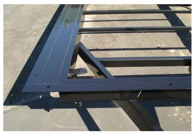
You can see large structural members on the perimeter, pre-drilled holes for connecting walls to the trailer frame, small interior structural members, and room for floor framing below trailer deck. The steel angles welded to the steel tube(s) forming the perimeter frame are great for placing the exterior walls on, but there is one negative tradeoff – plumbing drains must go through the floor adjacent to the exterior walls, not in the walls as they normally would.
