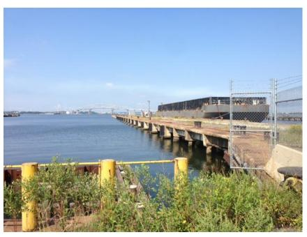
This image shows a finger pier extending out with a barge berthed on one side. There are large bollards and lighting, which indicates there is likely an electrical connection available shore side.
