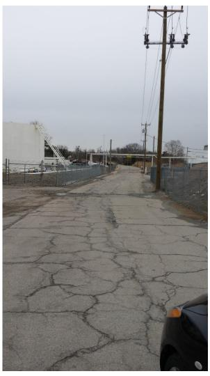
This image shows a site access roadway that is in poor shape and also shows an overhead restriction of a pipeline crossing up ahead that would require height limitations on traffic into and out of the site.
