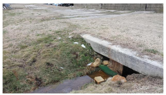
This image shows a stream/swale passing underneath a concrete structure, which indicates traffic passes over the bridge. The stream/swale has a wattle/sock and a steel grate over it, indicating there may have been debris blockages or environmental releases in the past.
