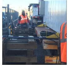
Hydraulic Jacks w/Teflon Sliding – Pushing Trays
