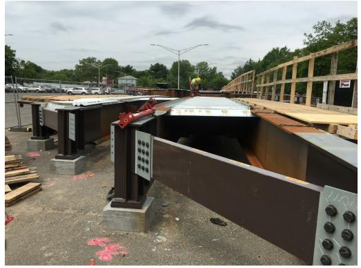
Stay-in-place (SIP) deck pans form the bottom of PBU slab
