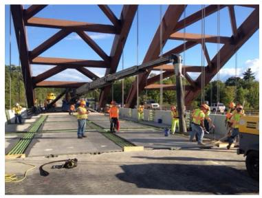
closure pour concrete being placed with telescoping conveyor truck
