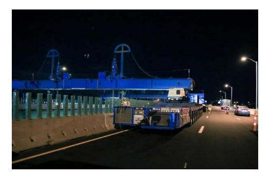
SPMT move median PBU span held with carrier beam and strand jacks
