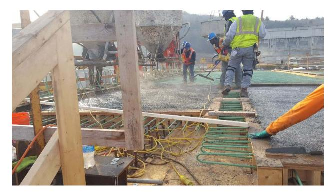
Before and during the concrete placement, quality control tests must be performed both at the plant for production and at the placement. Air content, temperature, and slump testing, plus the casting of concrete cylinders for laboratory compressive strength testing are the minimum tests needed to ensure a quality cast.
