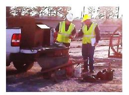
Quality Control Technicians reviewing Slump and Air Content tests To strike the deck to grade, the finishers will use a straight edge which probably rides the bulkhead forms to provide the unit's profile grade. The straight edge can be a roller screed or a vibratory air screed but depending on the quantity of concrete, a well
