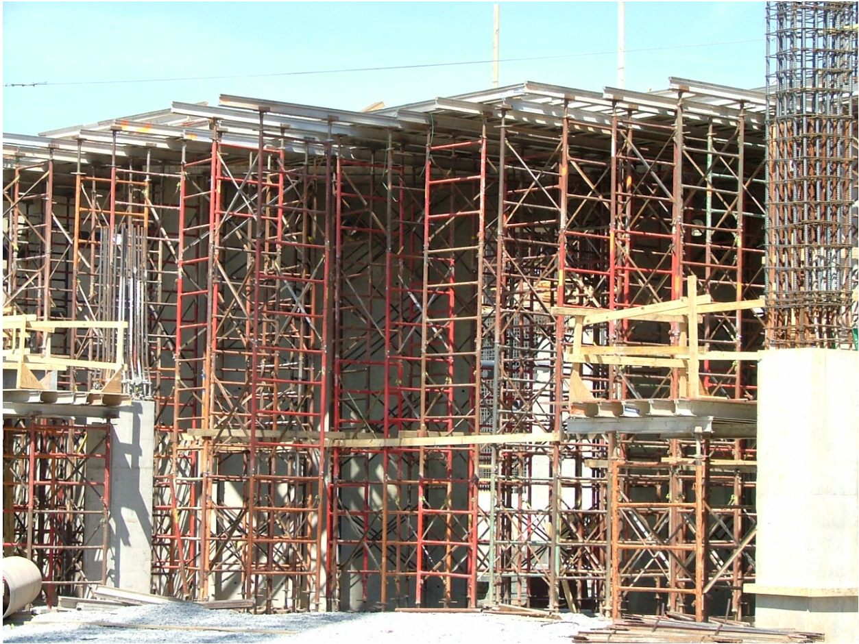
Figure 13. Example of sectional steel shoring towers with aluminum main beams and joists. (Photo courtesy of Aluma Systems.)
