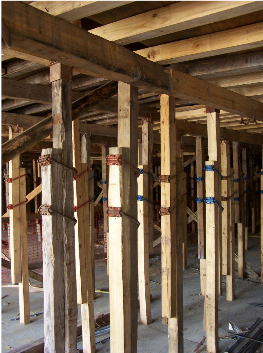
Figure 4. Timber formwork and shores using adjustable shore clamps.
