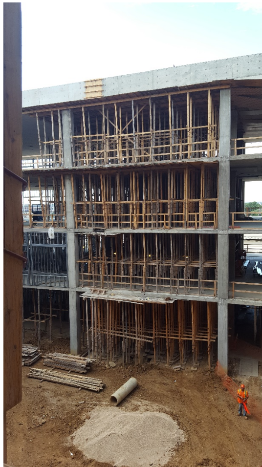
Figure 11. Timber backshores required due to pour strip.
