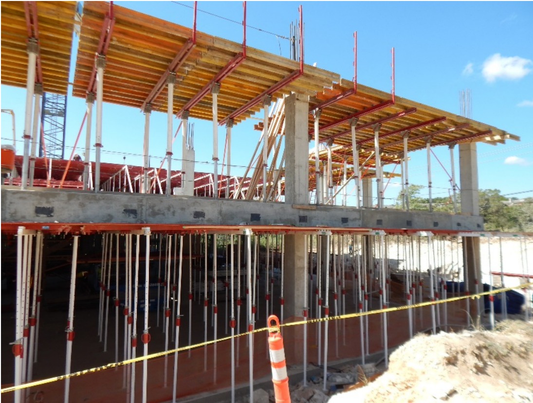
Figure 5. Proprietary shoring system. Proprietary systems commonly use steel or aluminum members and may also use timber for the horizontal members.
