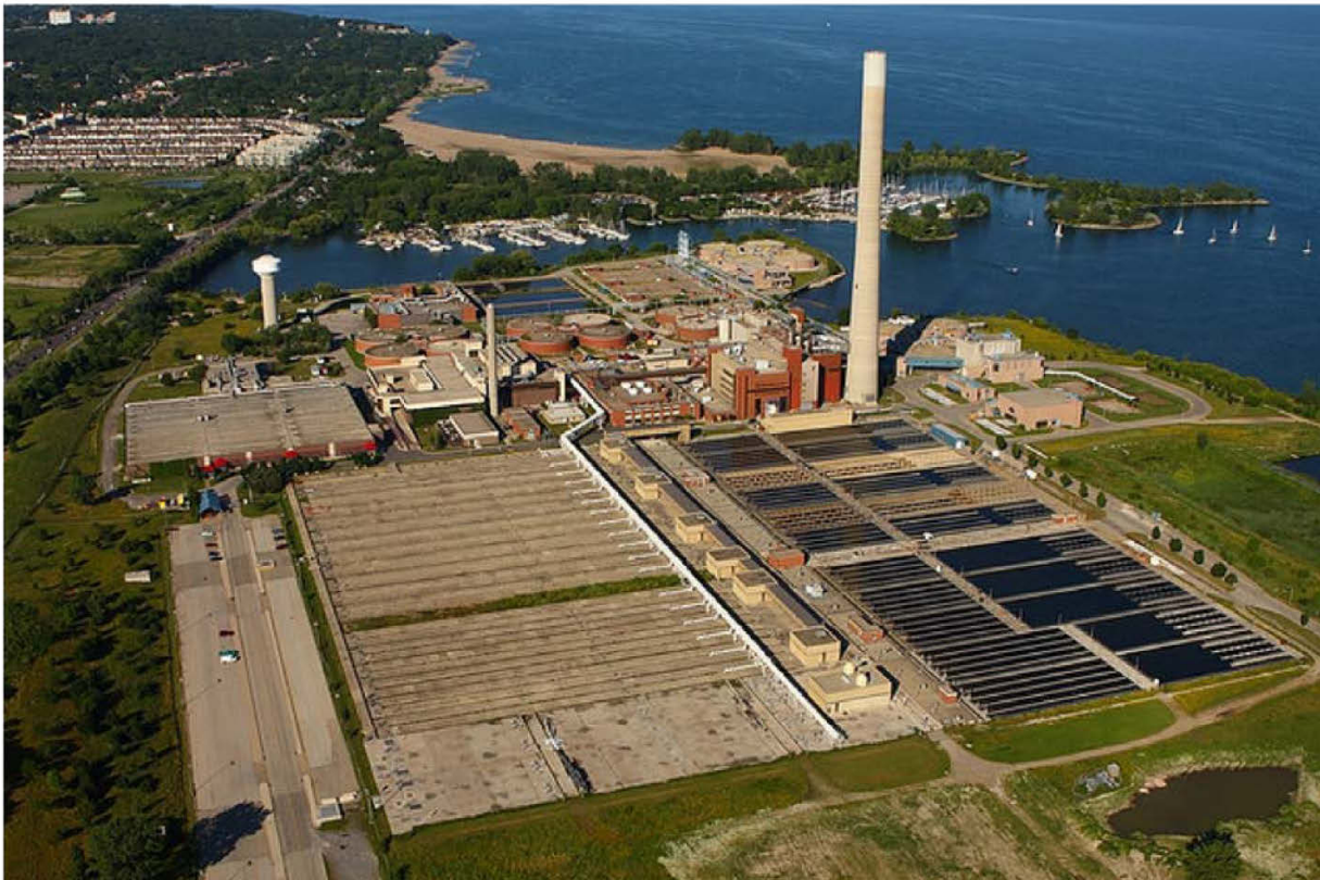
Figure 14 – Areal View of Ashbridges Bay Wastewater Treatment Plant
