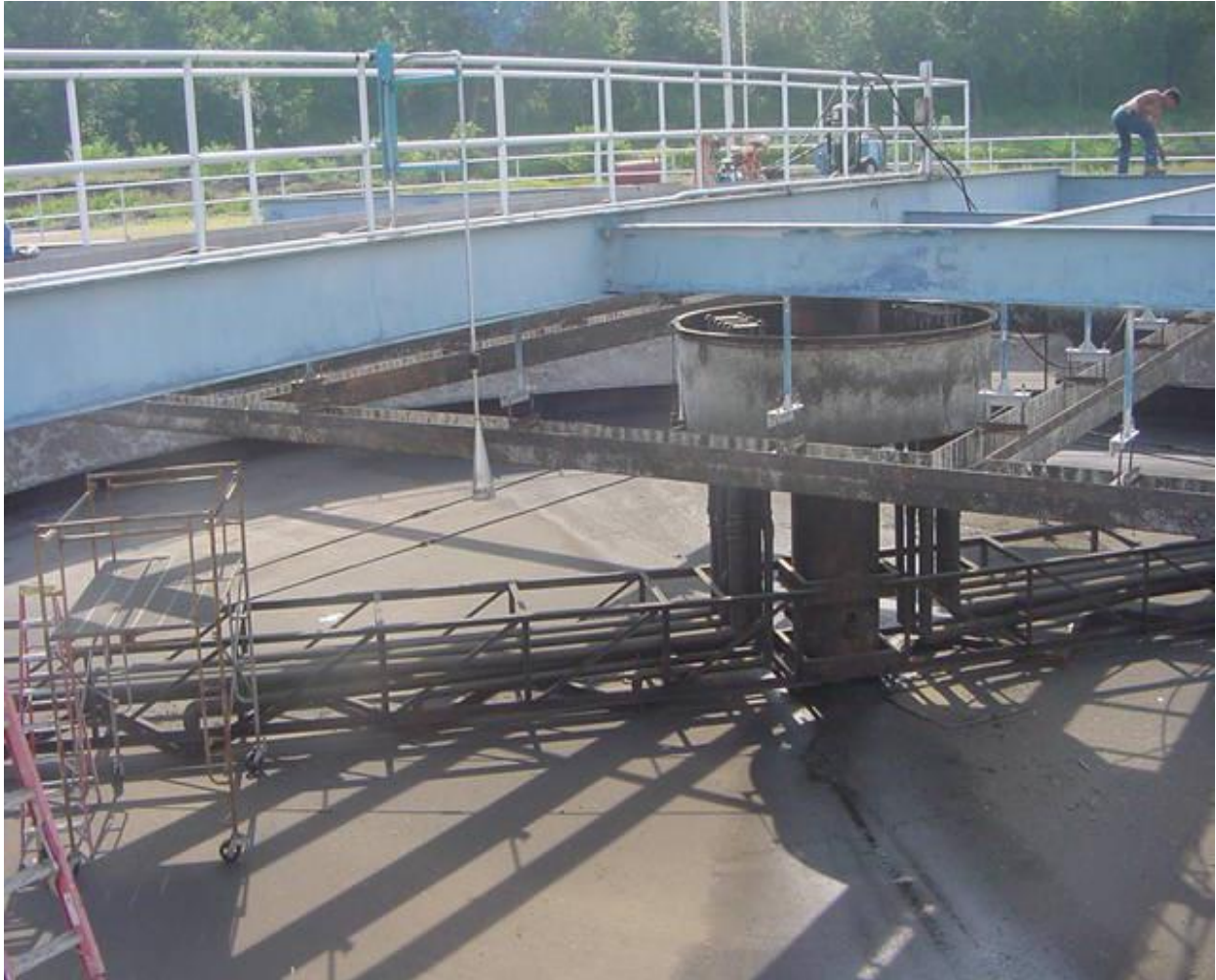
Figure 7 – Ultrasonic Sludge Blanket Level Detector
