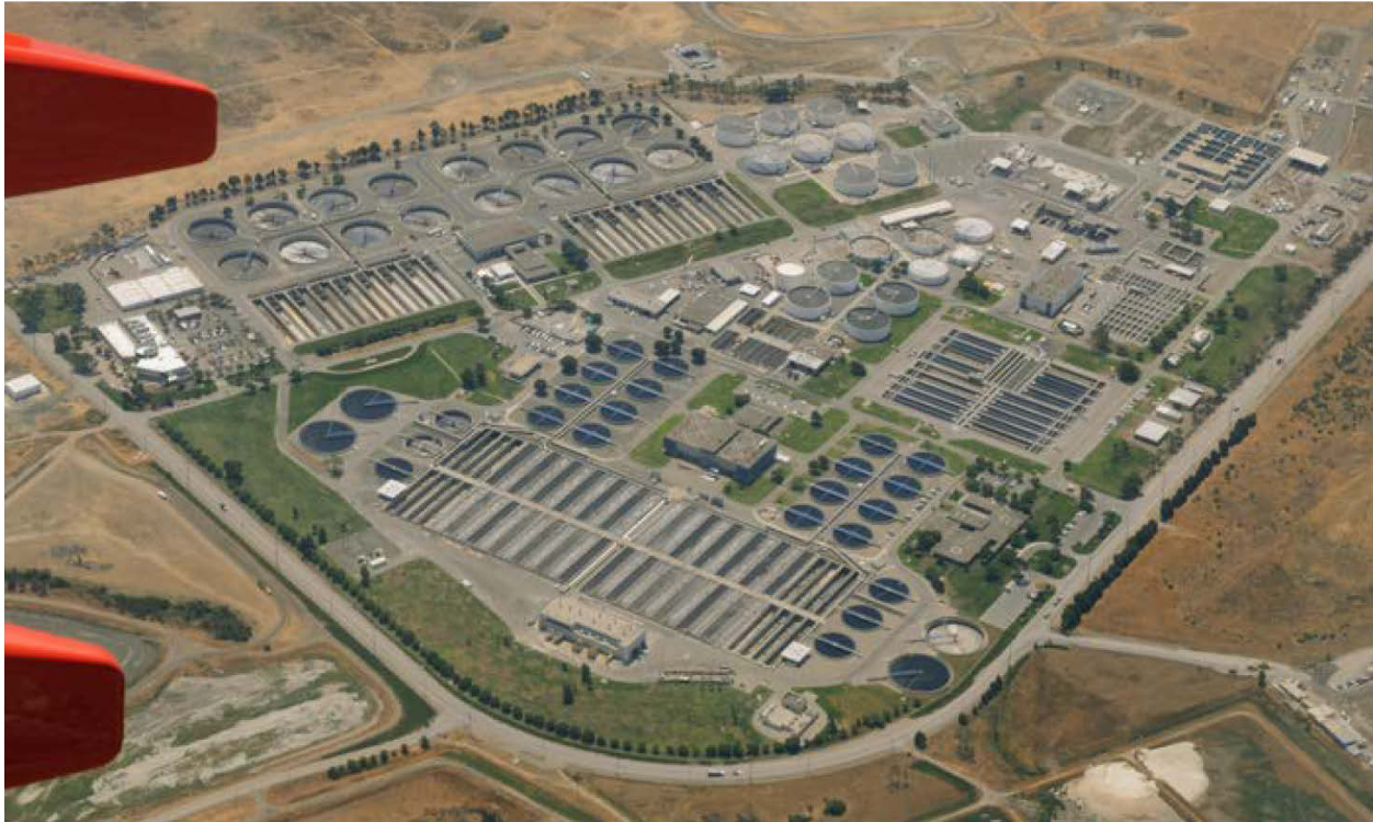
Figure 11 – Areal View of San Jose/Santa Clara Water Pollution Control Plant
