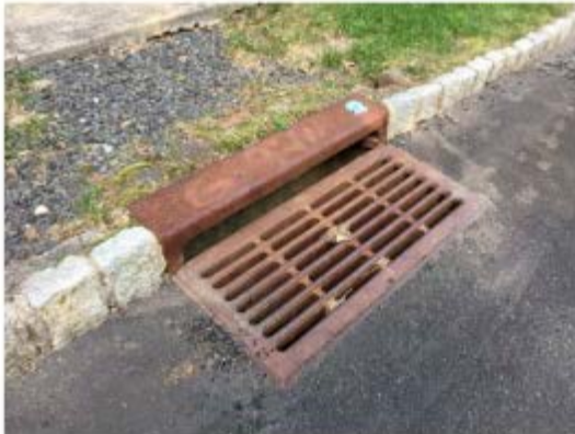
A cast iron grate cast iron curb inlet with "non-bicycle safe" grate
