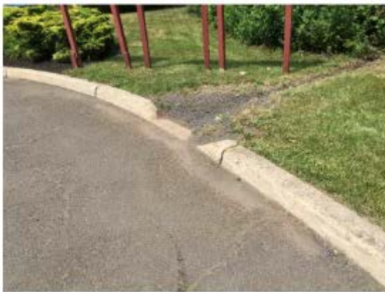
Simple curb cut for drainage
