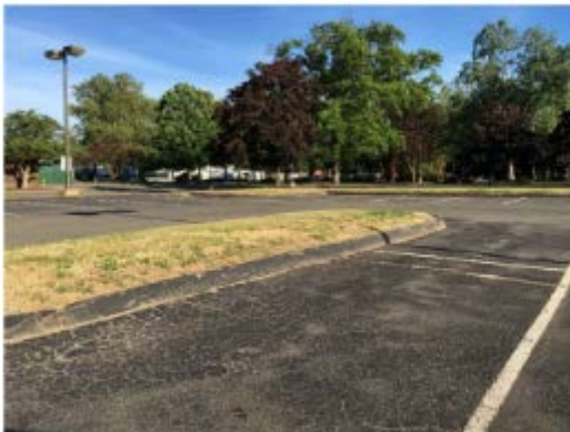
Asphalt Curb Island
