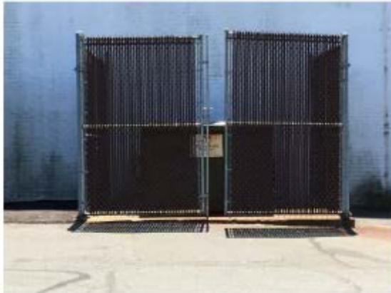
Chain Link Trash Enclosure with Vinyl Slats
