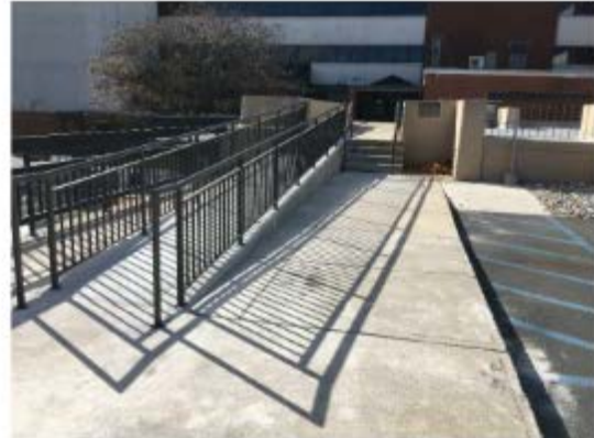
A concrete long ramp with hand rail
