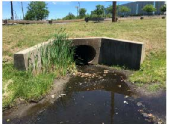
A headwall with wing walls
