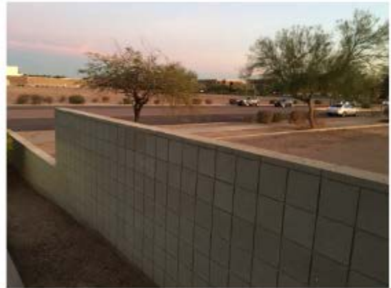
Concrete Screen Wall between adjacent lots
