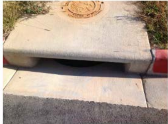
A concrete curb inlet in line with curb and gutter
