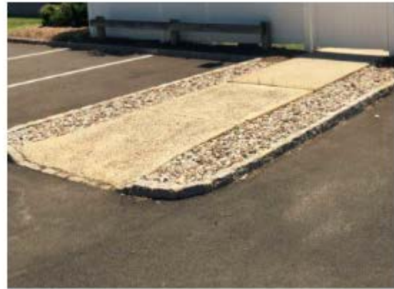
Belgium Block Curbed Peninsula with Sidewalk and Ramp
