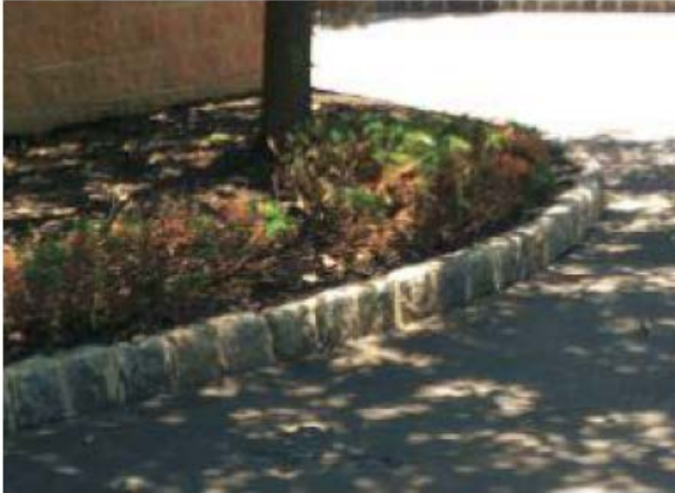
Belgium Block Curb on a radius
