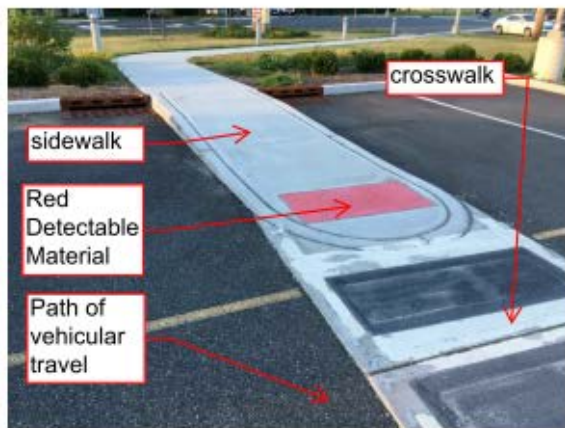
Detectable material at end of Peninsula sidewalk
