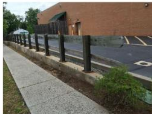
Small Concrete Retaining Wall with Timber Guide Rail at the Top
