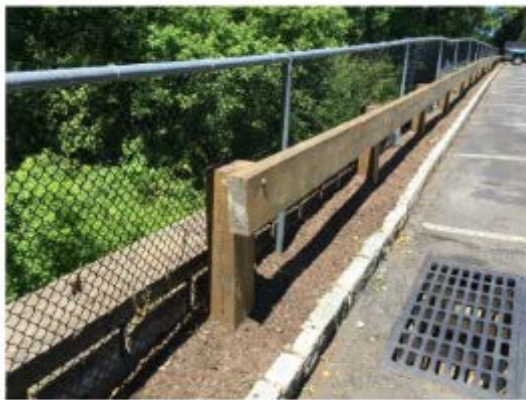
Timber guide rail on top of a retaining wall
