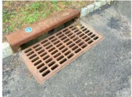
A cast iron grate cast iron curb inlet with bicycle safe grate
