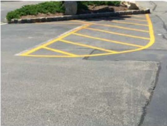
"Hybrid" Island partially striped for Truck Circulation Path
