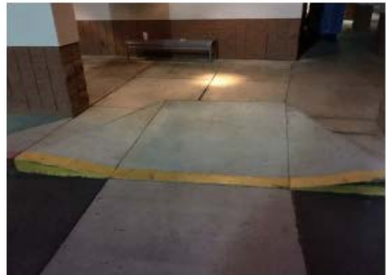
A Ramp with Detectable Finish scored in Concrete
