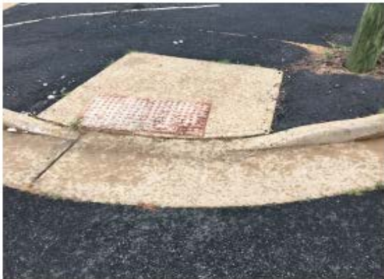
An Old Ramp With Detectable Material
