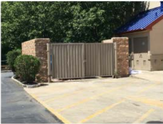
Block Trash Enclosure with Steel Gate
