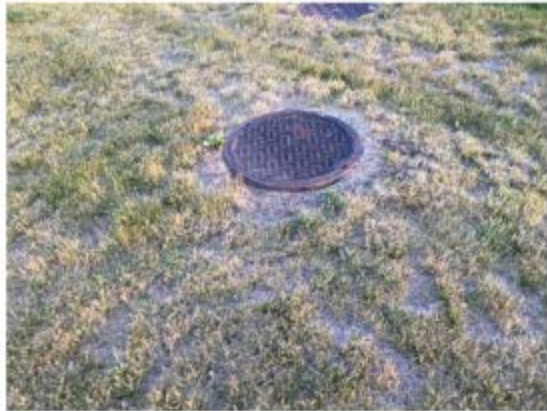
A manhole with a solid lid in a grassed area
