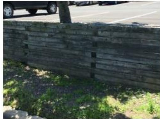
Timber Retaining Wall
