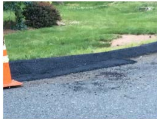
Asphalt Curb Repair
