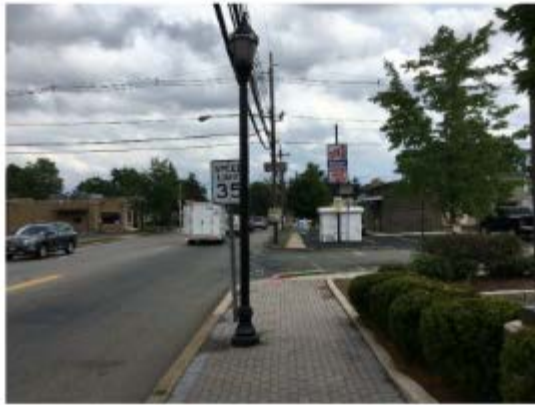
A Decorative Type Site Light on a Brick Paver sidewalk in the right of way
