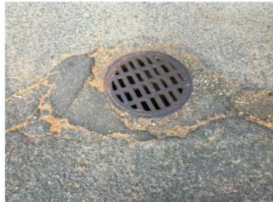
A manhole with a grated lid in a paved area
