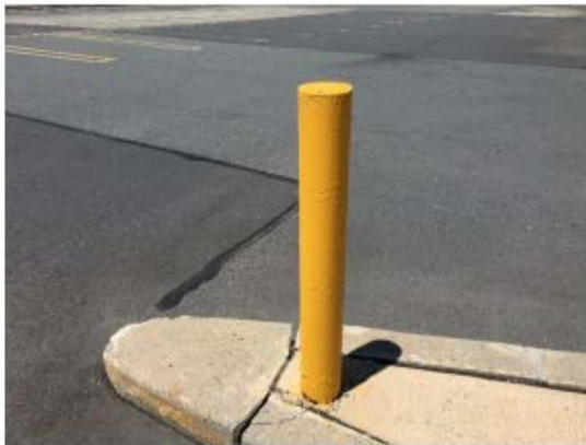
A painted, concrete filled, steel tube bollard
