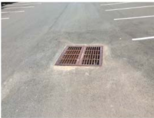
A double cast iron grate inlet flush to asphalt
