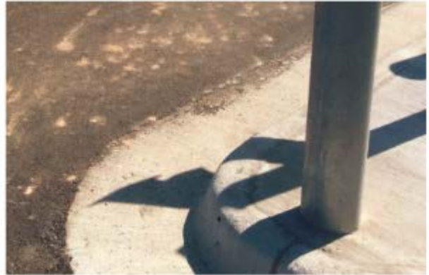
CURB AND GUTTER ON A RADIUS
