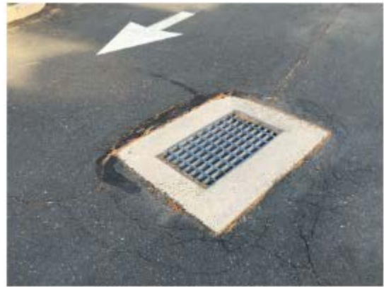
A single steel bar grate inlet, with concrete apron flush to asphalt
