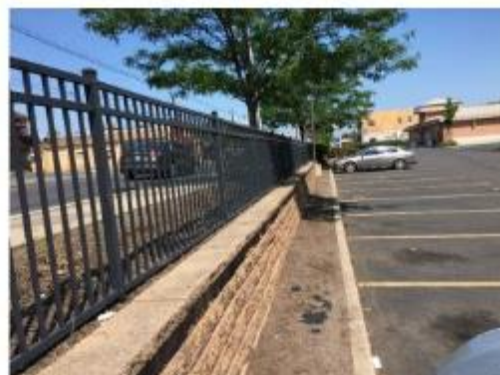
Modular Block Retaining Wall with Decorative Fence (Aluminum) at the Top
