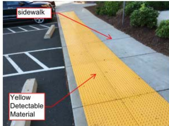
Detectable material along flush sidewalk edge
