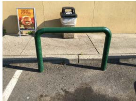
A steel tube "u-shaped" bollard protecting a storefront.
