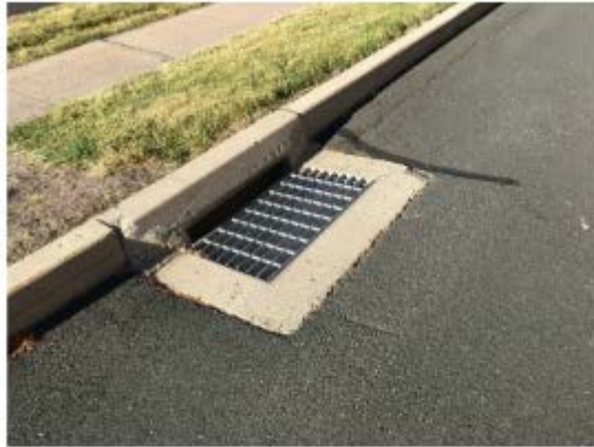
A concrete curb inlet with steel bar grate
