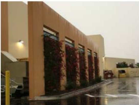
Vegetative Screen Wall in a loading area
