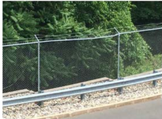
Chain Link Fence with Barbed Wire
