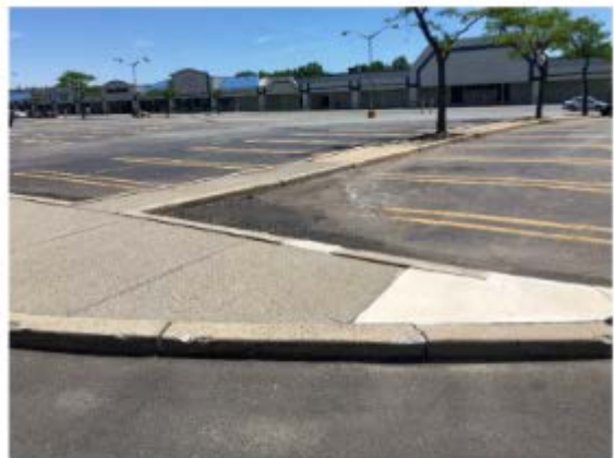
Concrete Filled End Cap with Concrete Longitudinal Island with Tree Openings
