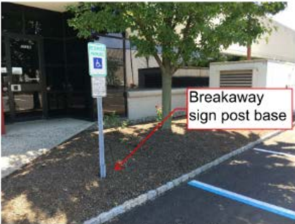
Reserved for Handicap Parking Sign with breakaway base
