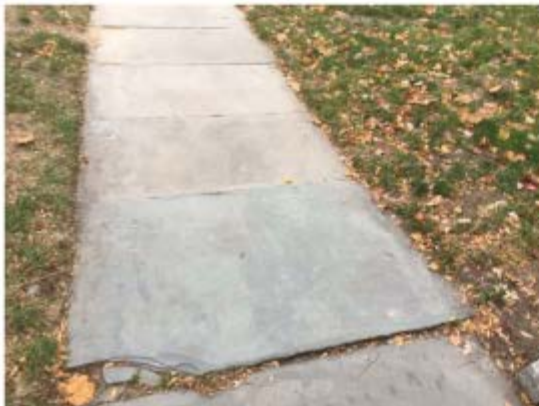
Slate stone Sidewalk
