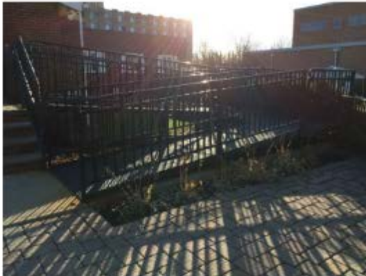
Long ramp constructed of steel
