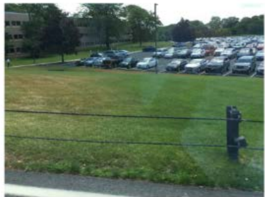
Steel cable style guide rail at the top of a hill
