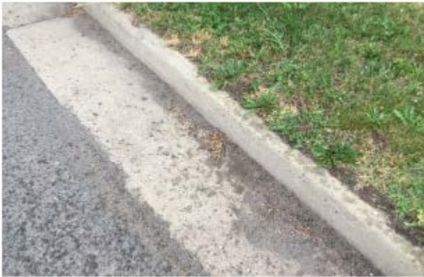
CURB AND GUTTER
