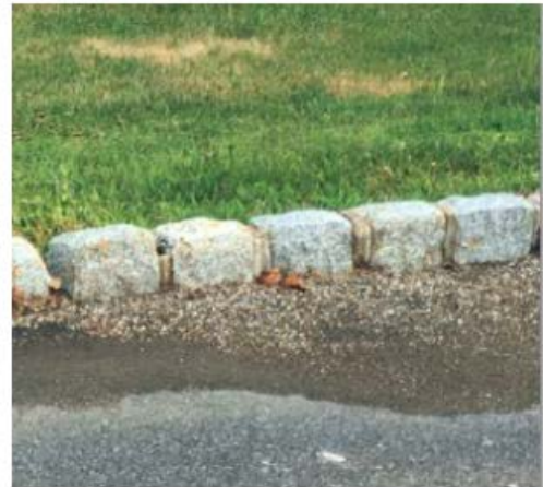
Straight section of Belgium Block Curb
