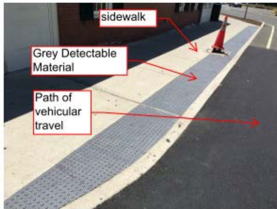
Detectable material along flush sidewalk edge
