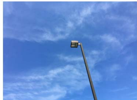
A Single Offset Mounted Showbox Type Site Light
