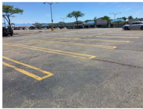
"U Shaped" Striping on 90 Degree Parking Spaces (2 Bays)
