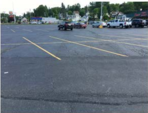
Angled Parking Spaces (2 Bays)
