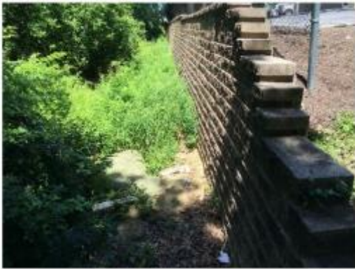
Modular Block Retaining Wall with Chain Link Fence at the Top
