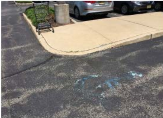
Ramp on a 45 degree to the sidewalk
