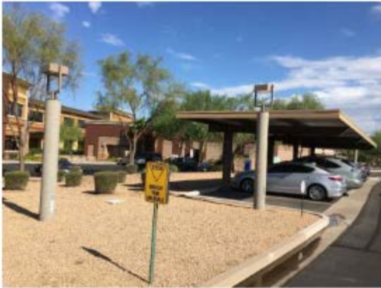
A Car Port / Covered parking structure
