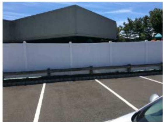
PVC / Vinyl Fence behind Timber Guiderail
