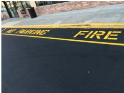
Fire Lane Striping
