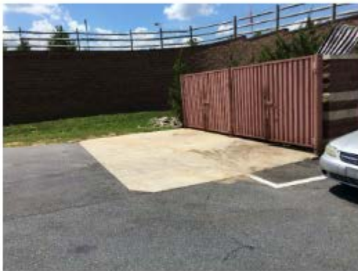
Double Wide Steel Gated Block Trash Enclosure with Concrete Apron
