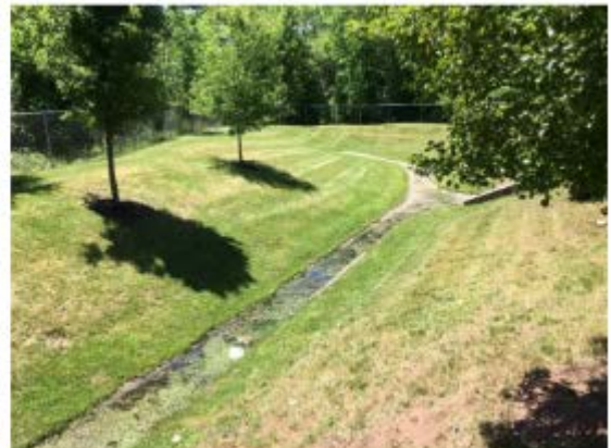
A detention basin with a low flow channel
