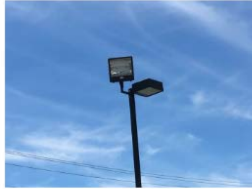
A Single Site Light with a second "flooding" fixture added, offset, angled and tilted
