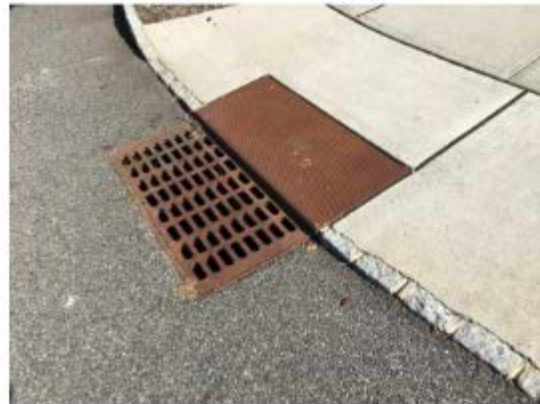
A cast iron grate curb inlet with mountable depressed curb / driveway apron piece
