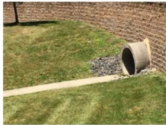
A pipe outfall through a retaining wall
