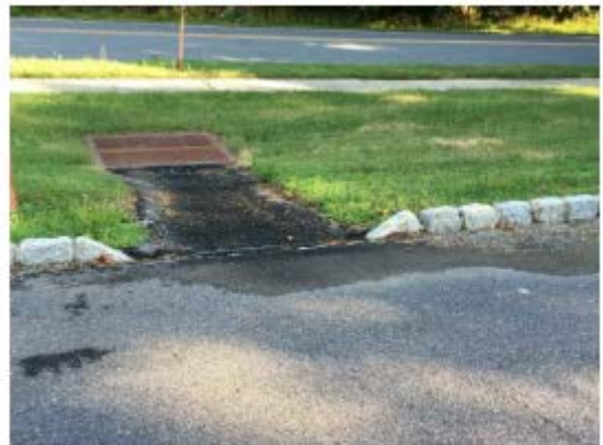
Curb Cut with asphalt flume to yard inlet
