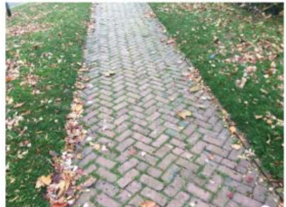
Brick paver Sidewalk
