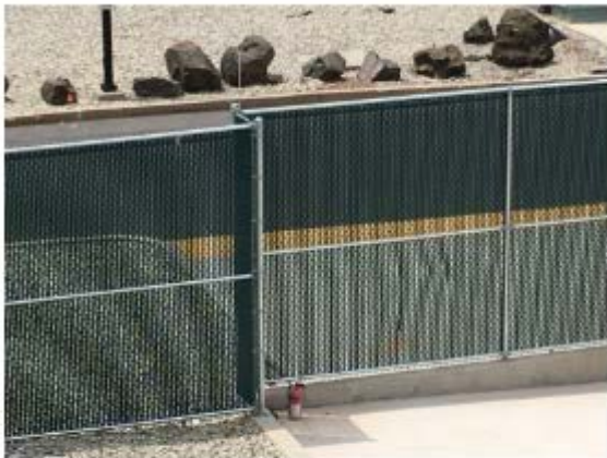
Chain Link Fence with Vertical Vinyl Slats
