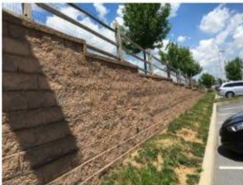
Modular Block Retaining Wall with Split Rail Fence at the Top
