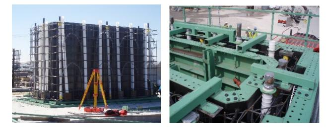
Vertical ductwork for a precast column segment prior to placing concrete in the cell
