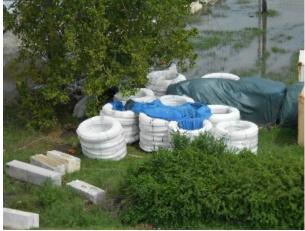
Flexible Plastic duct stored for placement
