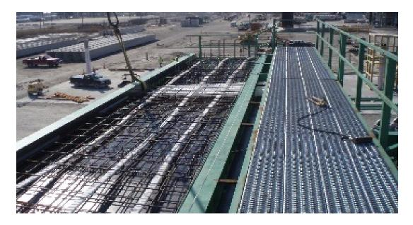
Transverse ductwork installed for a segment prior to placement of concrete in the cell
