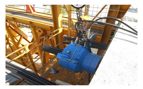
jacks. When the jacks reach the required pressure (compressive loads will be calculated in terms of hydraulic pressure in the jacks) the strands will be anchored in places with wedges to retain the loaded energy. The ducts are then pressure grouted to both protect the strand from corrosion and to permanently contain the stresses from the jacks.
