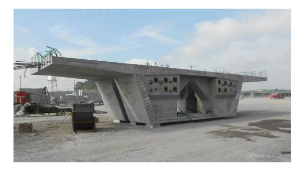
The above completed pier segment show anchor heads and metal ductwork in the cross-section face of the segment and shows transverse strands extending out the wings for stressing
