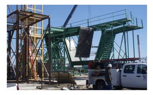
The interior form, or core form, provides the interior opening within the segment. The form supports the segment's interior top slab and controls the concrete thickness in the webs. For ease of stripping the forms after segment casting, the form sides should collapse and the whole system needs to travel in and out of the cell. In order to travel in
