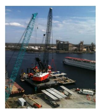
Gantries lifting segments using under wing straps with softeners at the concrete edges
