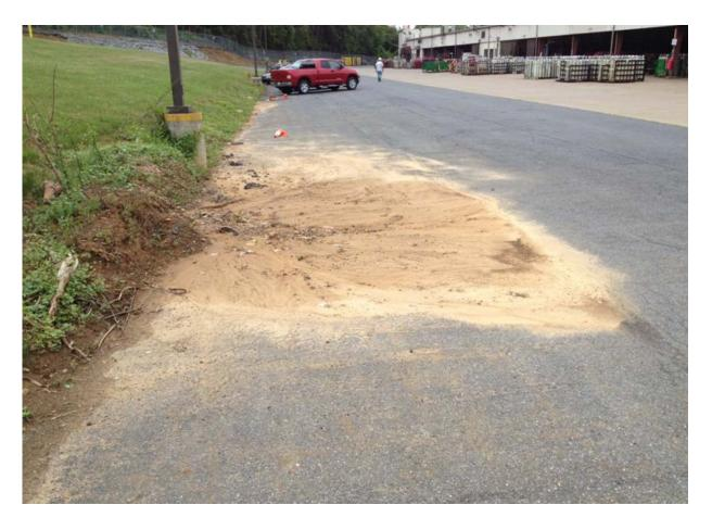
The soil erosion & sediment control plan should be designed to prevent erosion and sedimentation problems like the ones pictured above.
