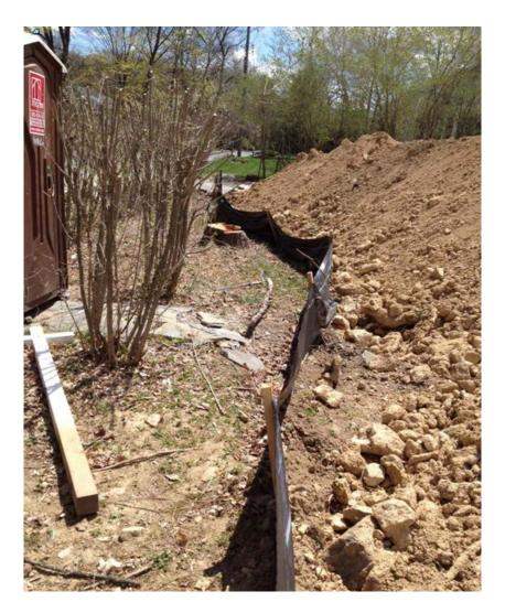
Staked hay bales and soil retention blankets can be used as substitutes for silt fencing. Soil retention blankets are biodegradable materials that can be used to protect disturbed areas or channels from erosion. The blankets consist of natural materials such as wood, straw, or coconut or else they are made from geotextile synthetic woven materials. Some typical specifications for each type of blanket are included below:
