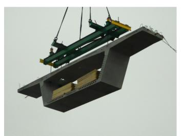
Crane lifting segments using picking frames and picking beams with anchors or sleeves cast into the top deck of the segment
