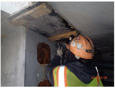
Forming span closure pours from interior of segment box
