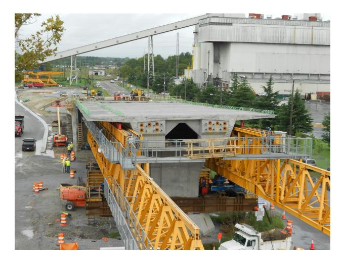
After the temporary supports are set to grade, inspected, and locked in their fixed position, the span is ready to start erecting segments. The first step is to load segments on to the supports (assume underslung truss for narrative) starting from one location and launch them longitudinally to their approximate location. Typically the segments
