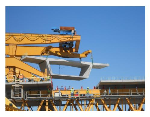
Gantries lifting segments using under wing straps with softeners at the concrete edges
