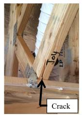
For this small truss, the hurricane clip can be reinstalled and connected to the scab members after the repair is complete.
