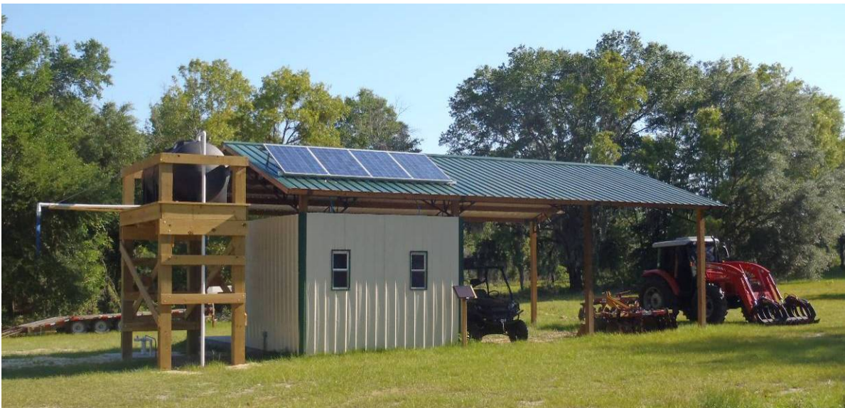
Figure 1 - An off-grid solar powered shop and fire fighting water well
