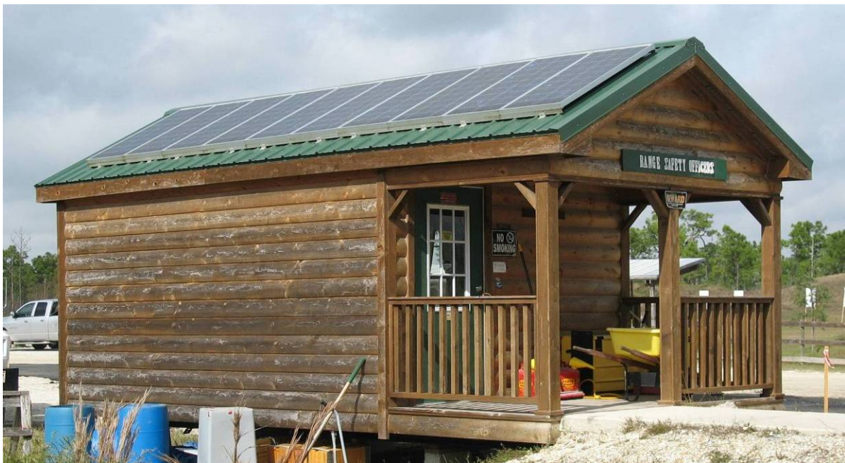
Figure 2 - An off-grid solar powered building in Punta Gorda, Florida
