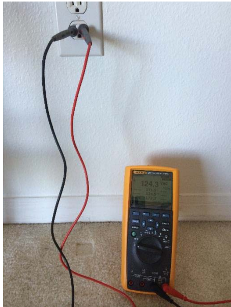
Figure 12 Hot to neutral voltage measurement
