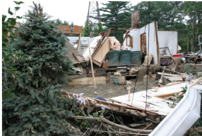
Natural gas explosion inside house, gas meter seen at foundation wall
