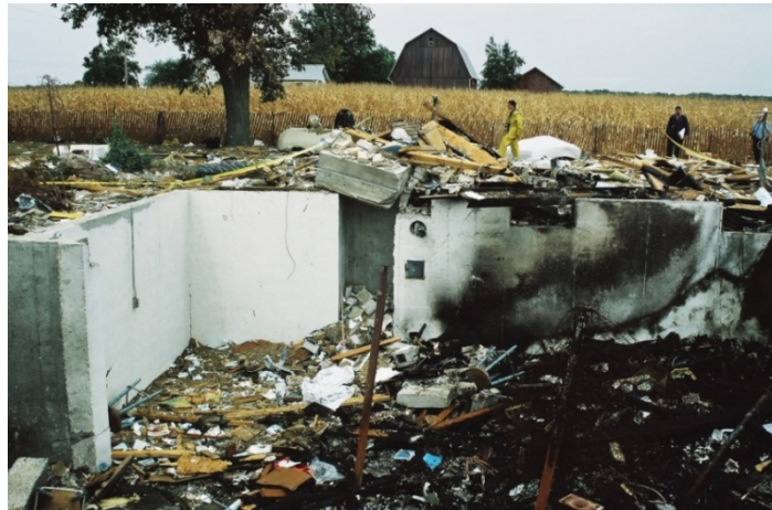
Propane explosion inside house, propane tank in background at top of photo
