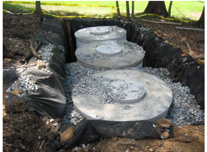
Recharge tanks installed with stone.
