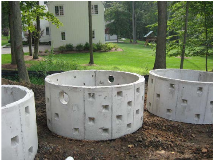
Recharge tanks awaiting placement.
