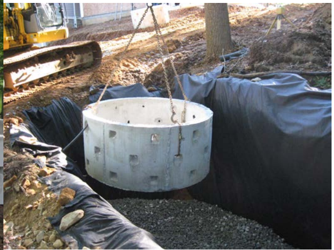
Recharge tank being installed. (Note filter fabric around stone).
