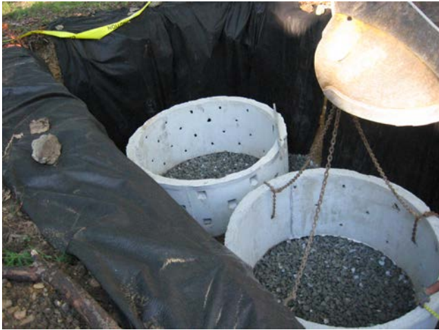
Recharge tanks placed within drywell.
