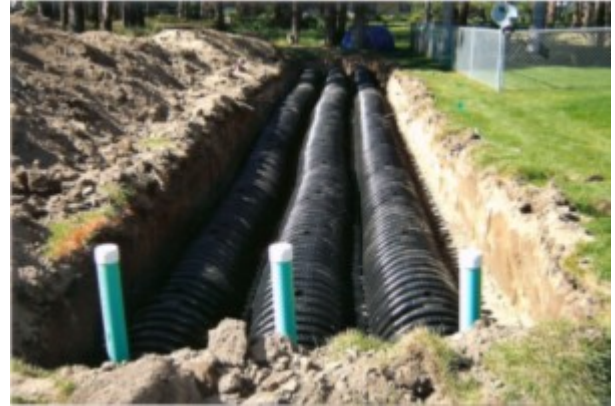
Infiltrator units placed in drywell.
