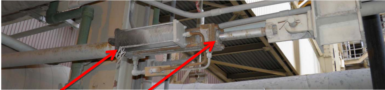
Shiny portion of piston indicates movement
