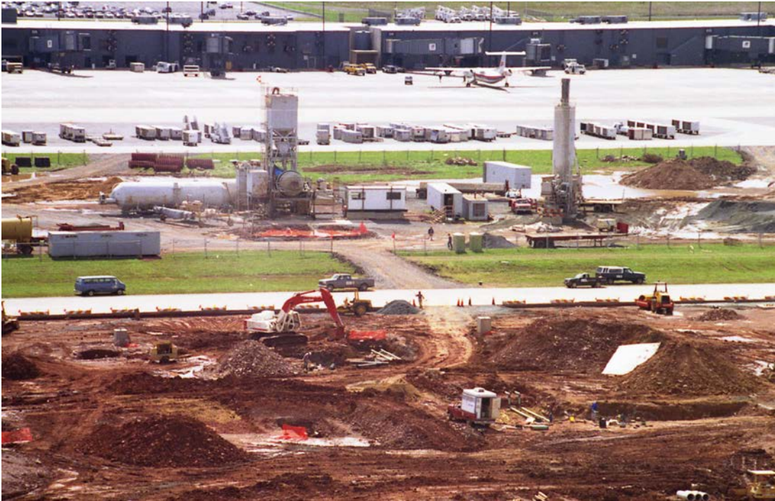
Central Drum Concrete Plant with extra cement storage next to a cement treated aggregate Pugmill Plant at an airport apron concrete paving site. Cement treated aggregate was used for base course material under 16" of concrete pavement.
