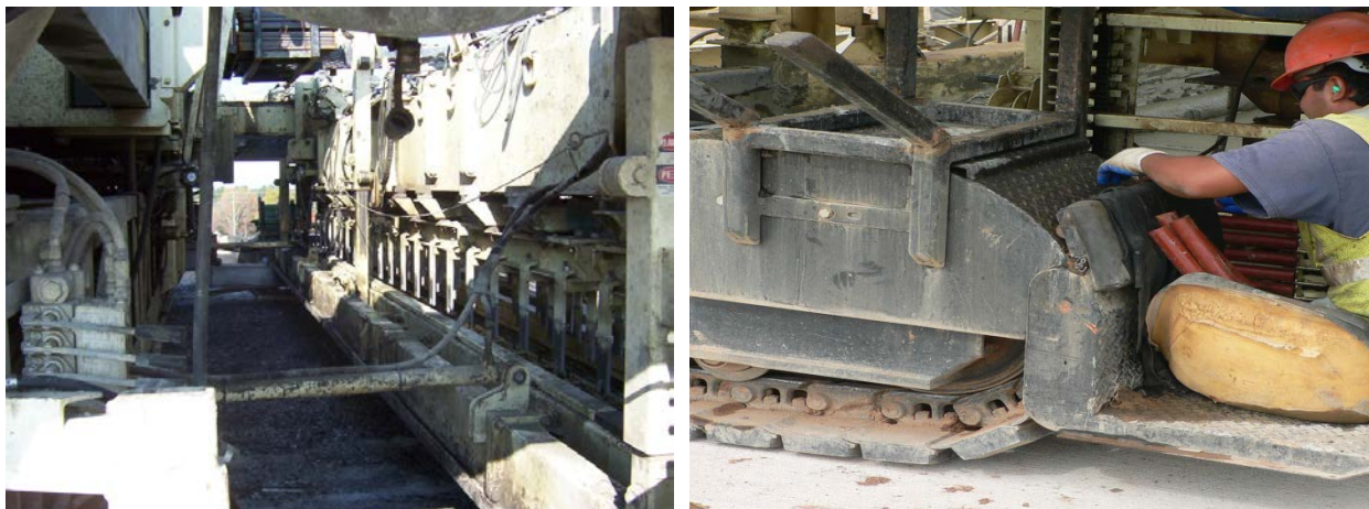
Concrete paving dowel bar inserter
