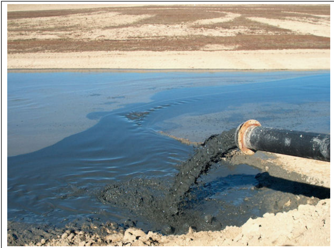
Figure 12b: – Typical discharge of silty material from pipe
