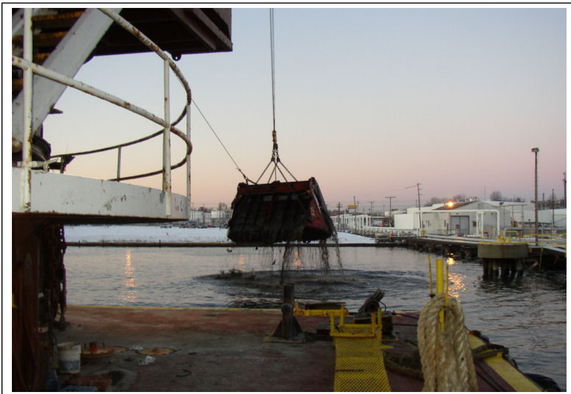
Figure 8a: An environmental clamshell bucket dredging soft mud in an industrial waterway
