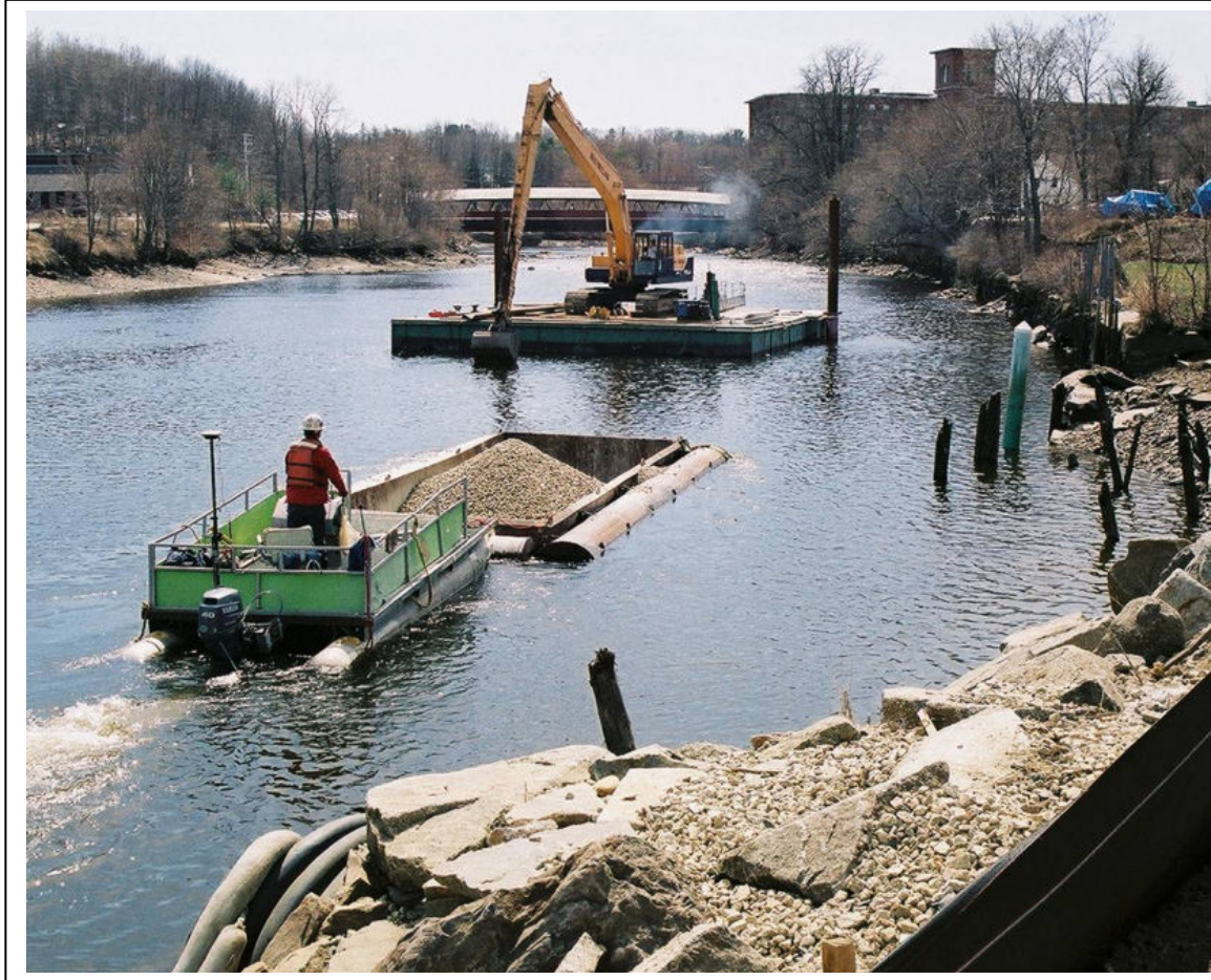
Figure 6b: 25 cubic yard, very small material barge; light draft about 2' – loaded draft about 4'
