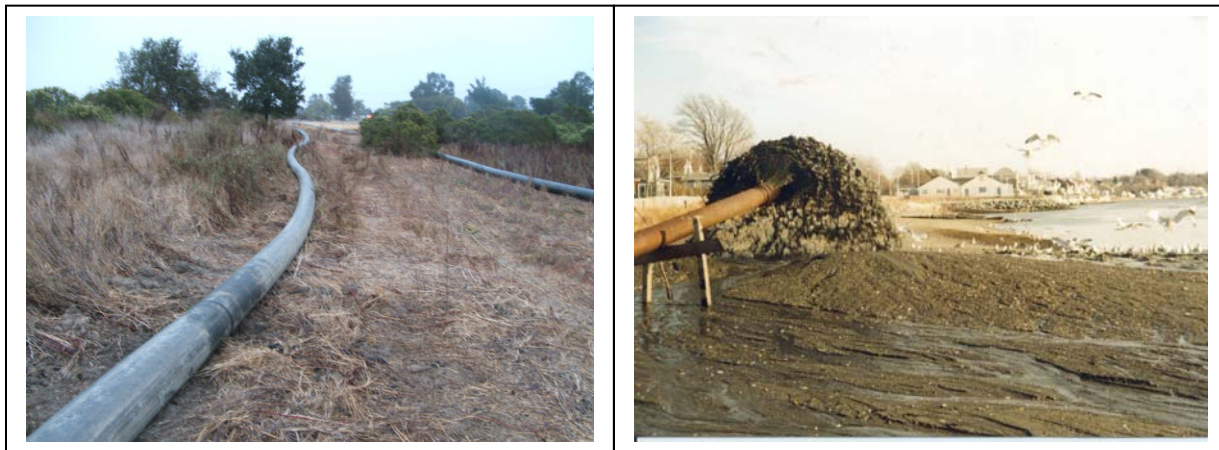
Figure 10: A 10” Dredge pipe routed through field (left) – 12” Dredge discharge on beach nourishment project (right)
