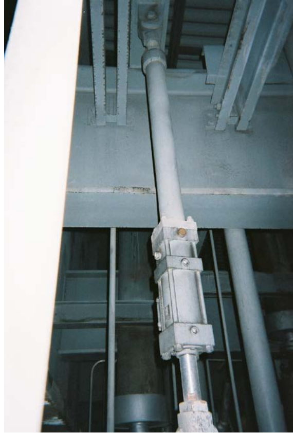
FIGURE 6.13 HYDRAULIC SNUBBER
