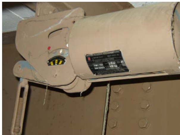
FIGURE 6.4 CONSTANT SUPPORT ROD HANGER. SUSPENDED FROM STEEL
