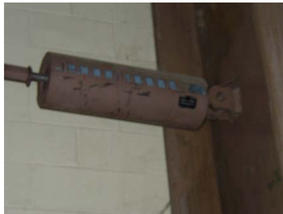
FIGURE 6.12 SWAY BRACE
