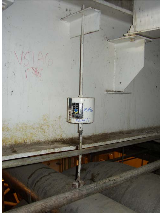
FIGURE 6.1 VARIABLE SPRING ROD HANGER
