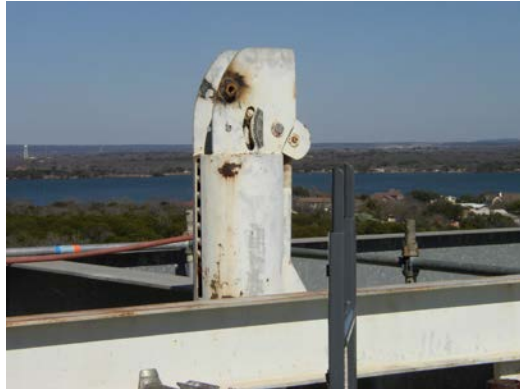
FIGURE 6.5 CONSTANT SUPORT ROD HANGER, RESTING ON STEEL
